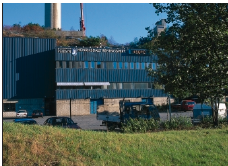
The Henriksdal waterworks in Stockholm ensures state-of-the-art, efficient removal of phosphorus and nitrogen.
