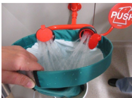
Figure 4 Testing Eyewash station
