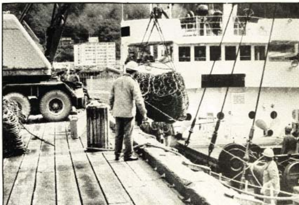
Once off-loaded in Alaska, the 22,000-pound torpedonet were to be used to prevent erosion on river banks near fishing villages.
