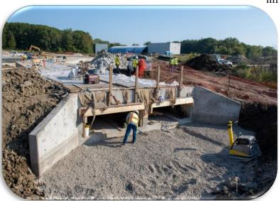
Photo LBNF site preparation work. A 500-foot-long box culvert was constructed to redirect Indian Creek to flow under a portion of new permanent hill needed for the project. The culvert includes a naturalized channel for fish. Photo: Ryan Postel, Fermilab
