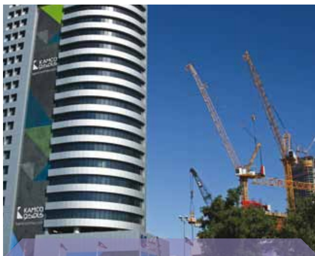
Kuwait City: skyscraper under construction.
