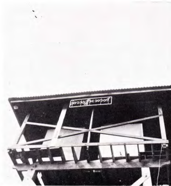
Fig. 10. The recently erected neon sign in Mon indicating the name of the temple
