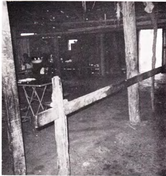
Fig. 3. The section set aside for buffaloes in a house, in which the earthen floor can be clearly distinguished
