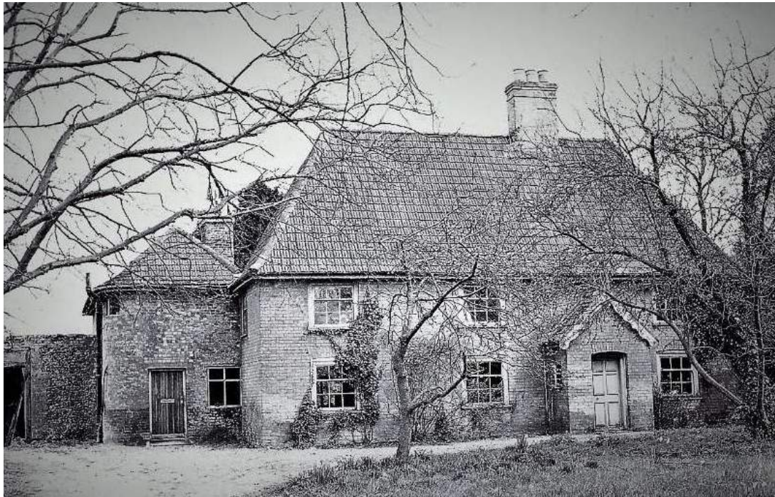
Maltings Farm before demolition c.1970 Photograph H Wood
