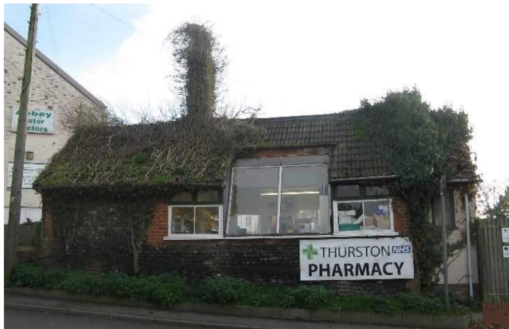
Thurston Pharmacy 2015 established in the Granary's grain quality inspection office
