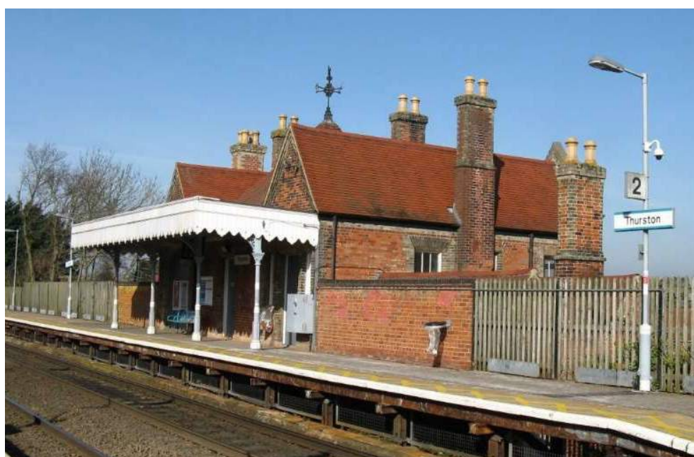
Thurston Station, the present unmanned halt 2017
