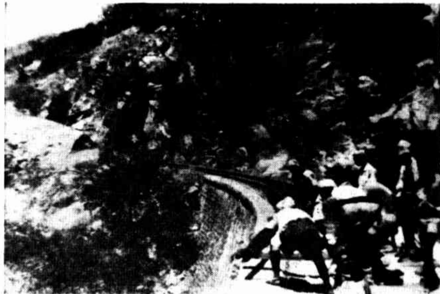
Guerrillas of the Eritrean Liberation Front, who are in revolt against the Ethiopian regime of Emperor Haile Selassie, tear up railway tracks on a bridge spanning a deep ravine on the line between Keren and Asmara in Ethiopia. This is one of a series of photographs taken by a Syrian photographer, Ahmad Abu Sada, who says he has spent a month with the guerrillas. — AAP-AP cable picture.
