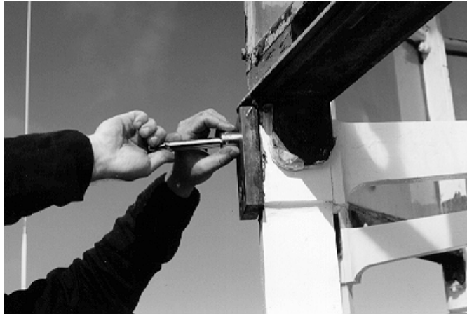
Figure 38. To provide a plumb mounting surface for the gallery deck, each mounting surface was covered with Belzona (a two-part metal paste); then the mounting plates were installed and tightened until they were plumb. The excess Belzona can be seen oozing near the middle of the plate.
