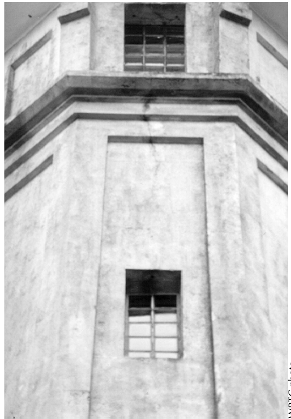
Figure 10. Cracks like the one here, extending down from the belt course of this concrete lighthouse, should be monitored for movement before any patching is performed.
