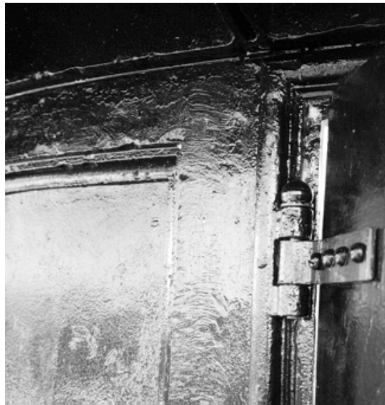
Figures 36 and 37. The left image shows the condition of the iron exterior service room wall before rehabilitation. The right image shows the same area after power hand tool cleaning and coating. The crescent shaped scars in the iron are from the arc of a grinding wheel.
