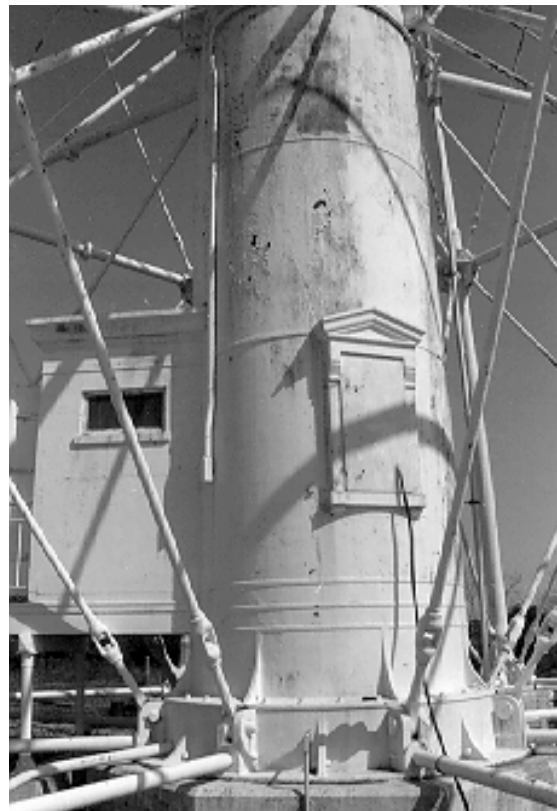
Figure 27. Blistering paint, as pictured here, should be removed and the affected areas properly primed and painted.
