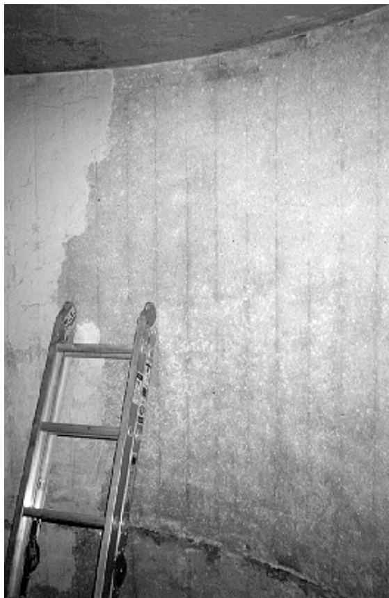
Figure 24. The interior paint was effectively removed using needle gun scalers, without damaging the concrete as evidenced by the visible impressions of the formwork boards.
