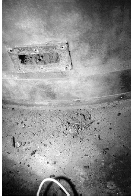
Figure 20 (above). The finished vent installation: 15-lb. roofing felt was placed between the bronze vent grill and the cast-iron parapet wall.
