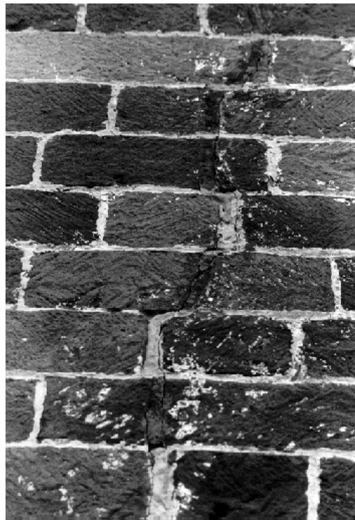
Figure 15. Cracks such as these in a sandstone lighthouse should be monitored for movement prior to treatment.
