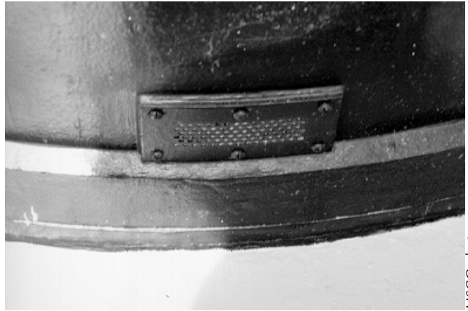
Figure 19 (left). Buildup of rust in parapet wall vents.
