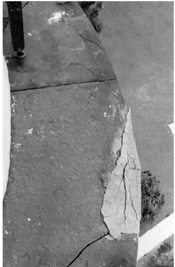
Figure 22. A failing repair made to a stone gallery deck using a simulated stone material. A stone dutchman repair should have been used.
