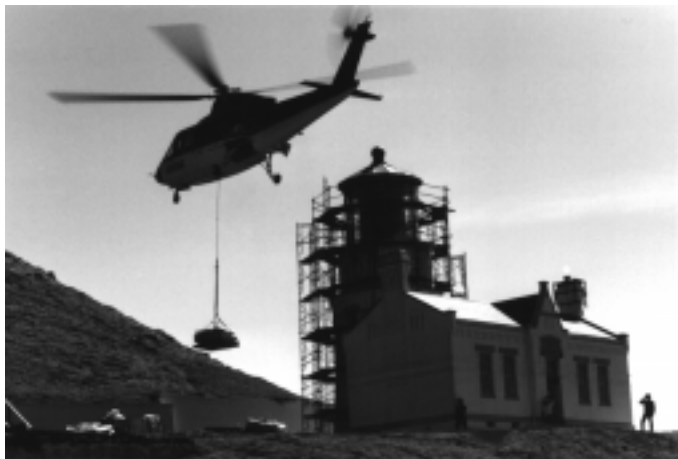
Figure 45. Staging the work. Note the temporary location of the auxiliary light on the fog signal building chimney.
