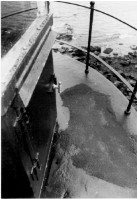
Figure 7. Ponding is occurring on this gallery deck near the base of the lantern parapet wall. This ponding has led to an active leak that occurs even during light rain conditions. A condition such as this should be remedied before the mothballing period.
