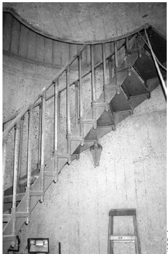
Figure 25. After the cast-iron stairs were blast-cleaned, they were rinsed to remove all traces of lead dust; flash rust immediately formed (as seen in this photo). Before painting, this light rust was removed with wire brushes.
