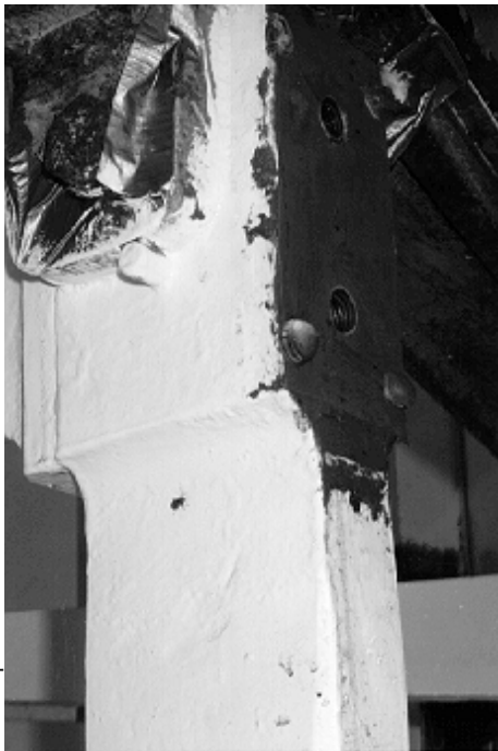
Figure 39 (left). View of the mounting surface after the Belzona had cured and the mounting plate had been removed. The 'knobs' or protrusions on the surface are where the Belzona was squeezed through the holes in the mounting plate. These were ground off along with the excess Belzona that squeezed out around the plate.
