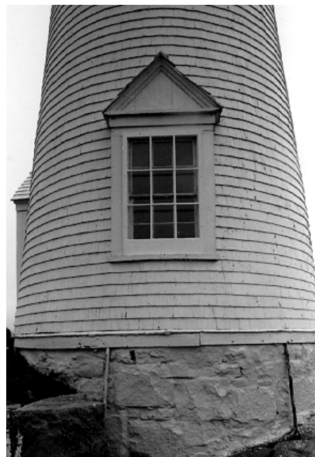
Figure 2. Stone masonry foundation in a 38-foot-tall wood-frame lighthouse in Maine.
