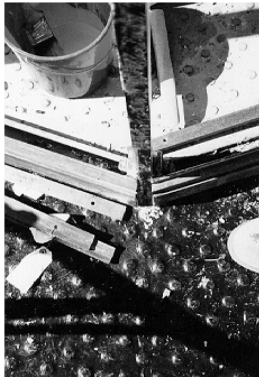
Figure 12. Detail of the bronze sill when the lower mullion is removed; the fastener is re-tapped and the cast-iron column is treated with a rust converter. Note that the bronze astragals have been cleaned and are ready to accept the glazing system.
