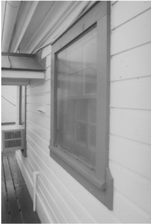
Figure 13. This image shows a Class I paint condition: virtually no deterioration, only some soiling and possible salt buildup resulting from the open-water location of the lighthouse.
