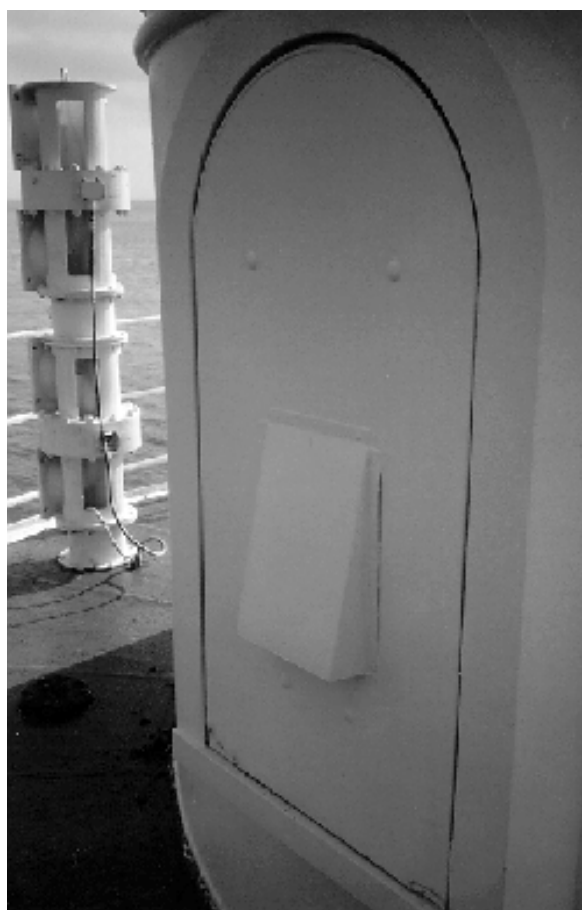
Figure 4. A good example of a blocked window using a metal panel fitted with a hooded vent. For more adequate ventilation, the vent should be larger.
