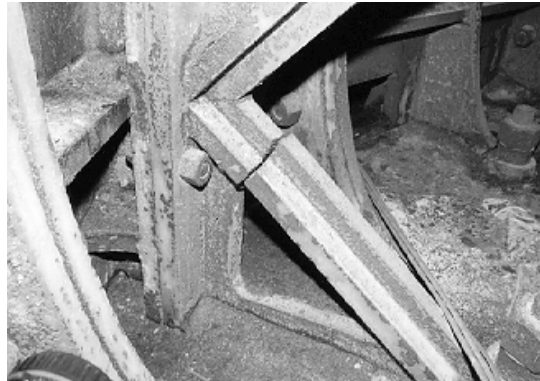
Figure 18. The internal structural skeleton of this lighthouse is cracked because of overloading possibly during assembly.
