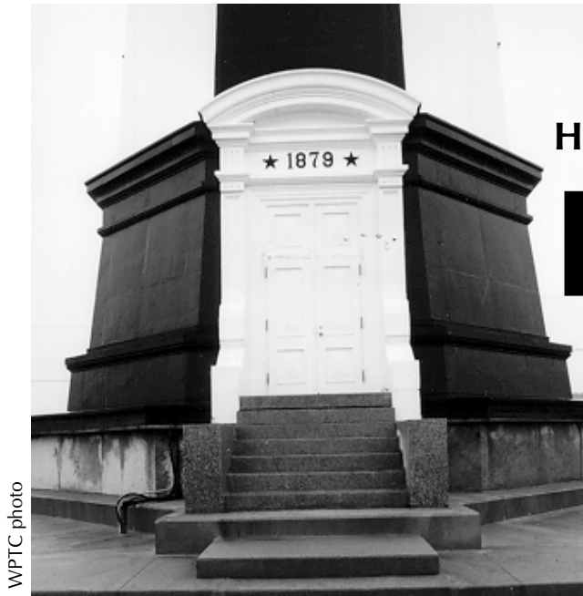
Figure 1. Close-up of large, double-leaf, wood-frame and panel doors at the Cape Henry Lighthouse (second tower), Fort Story, Virginia.
