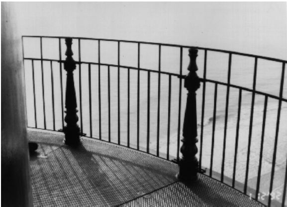
Figure 15. A replica handrail is installed.
