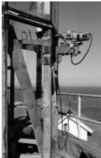
Figure 35. Jig used to bore holes in the gallery bracket tenons.
