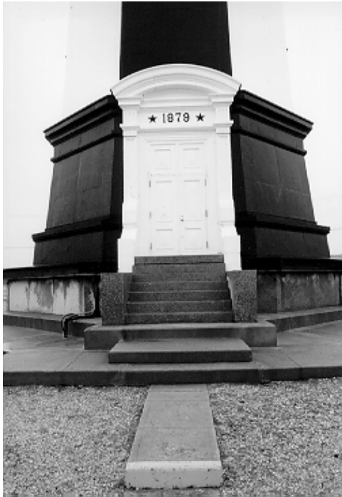
Figure 8. An example of the level of detail achieved with cast-iron construction.
