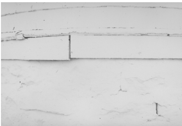
Figure 11. Open joints like those between these skirt boards must be properly primed, painted, and filled before mothballing the lighthouse.
