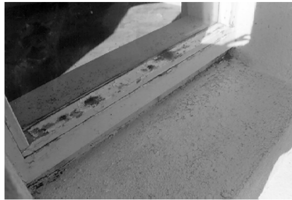
Figure 26. This steel casement window frame was not sealed properly and as a result has begun rusting from the inside out.
