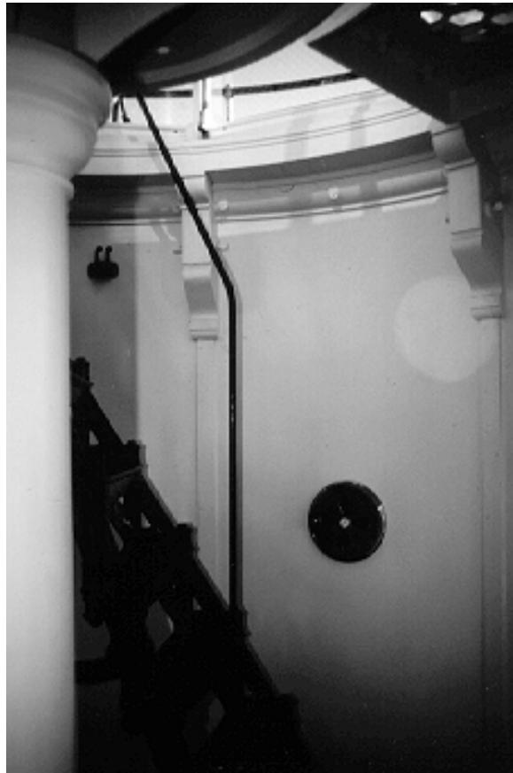
Figure 38. Service room bracket after chemical cleaning.
