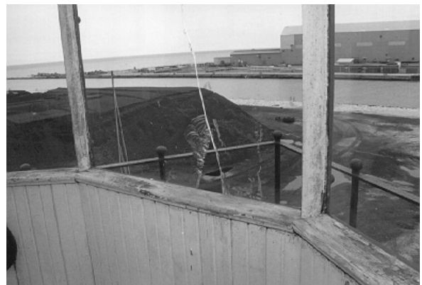
Figure 5. Storm glass with holes should be replaced as soon as possible to minimize water infiltration. If immediate replacement is not an option, the storm glass can be temporarily patched.
