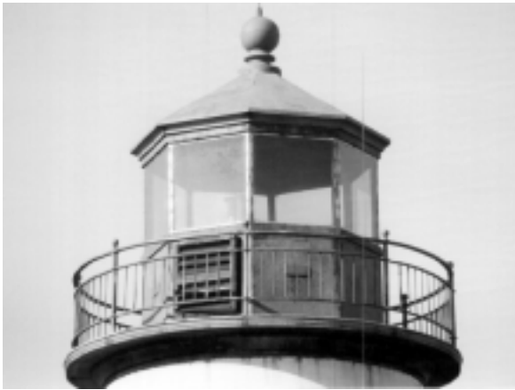
Figure 4. Close-up of the fourth-order lantern at Coquille River Lighthouse in Oregon.
