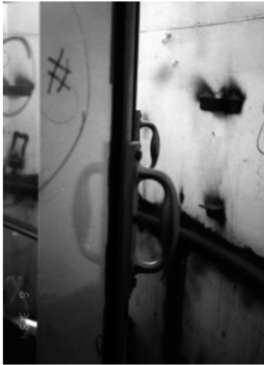
Figure 8. New hand holds were replicated to replace missing pieces. These exactly match the originals.
