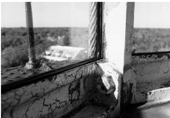
Figure 16. This detail shows the new glazing system in place with associated cast-iron post and bronze sill available to receive additional cleaning and paint removal.
