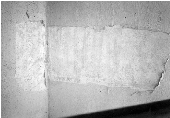
Figure 23. The water-based paint stripper was very effective in removing the many layers of paint from the exterior of the tower.
