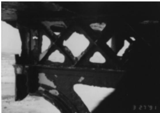
Figure 12. Some brackets were so deteriorated that they were totally exposed to the elements.
