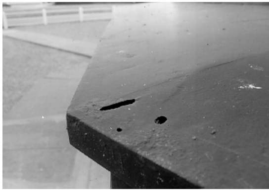
Figure 12. Close-up of localized corrosion or pitting where the corrosion has eaten through the cast iron.
