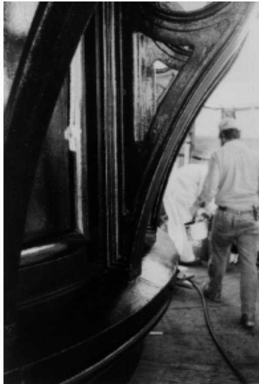
Figure 17. The cast-iron belt courses are repinned to new masonry beneath.
