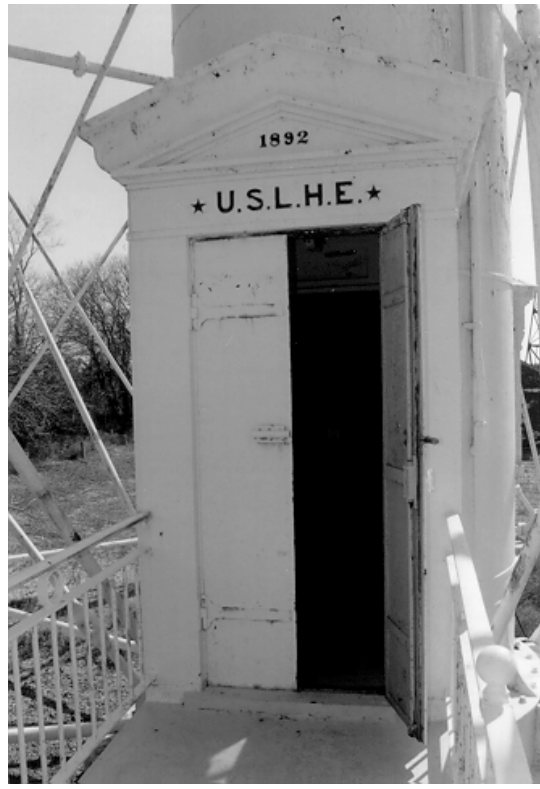
Figure 6. Close-up of the neoclassical, double-leaf, sheet-iron door at the Cape Charles Lighthouse, Smith Island, Virginia.
