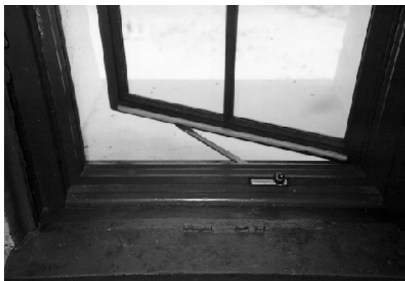
Figure 10. Close-up of a recently restored replacement metal window at Cape Hatteras Lighthouse. Now that the repair work is done, all that this window needs is the hardware lubricated and periodic maintenance to remain in operable condition for the next 50 years. At the time of this lighthouse restoration, it was discovered that the original windows were not repairable and funds were not available to replicate the original cast-iron frame design. The original windows were more like a shutter, constructed in two parts, hinged at both sides and meeting in the middle. The new landing windows were installed as a temporary measure until additional funds are available.
