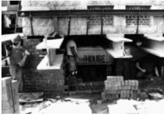
Figure 22. Construction of a new foundation around the support beams.
