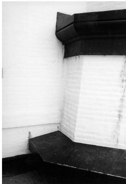
Figure 41 (left). This masonry lighthouse has been detailed with a two-tier cast-iron water table (the iron portions are painted black). Rust-bleed is occurring along lower edge of the upper tier.
