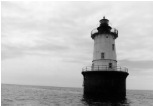
Figure 3. Example of an all-cast-iron construction "sparkplug" caisson-style lighthouse.
