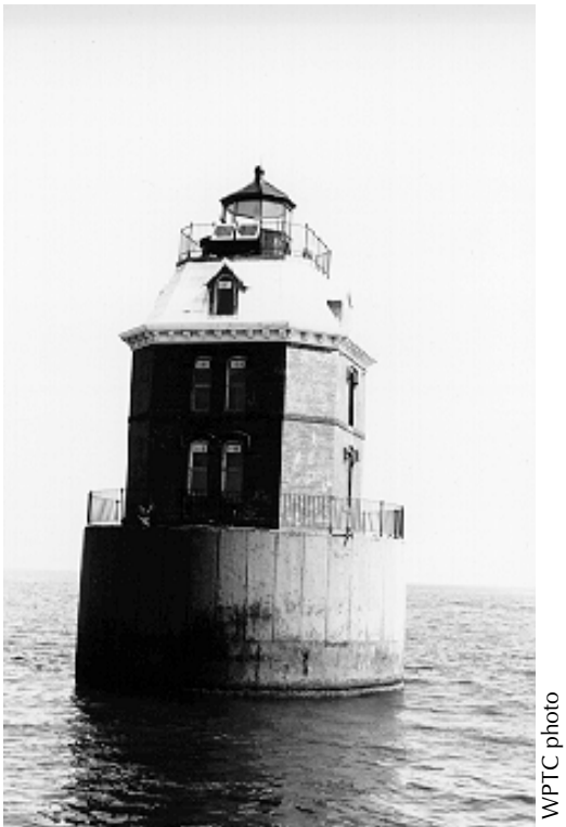
Figure 3. For the construction of this caisson-style lighthouse, unreinforced concrete was used as ballast to sink the cast-iron caisson foundation deep into the mud on the bottom of the Chesapeake Bay in Maryland.
