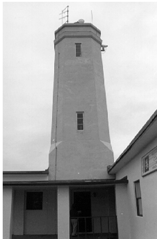
Figure 5. St. John's River Lighthouse, Mayport, Florida, was constructed of reinforced concrete for its economy and low maintenance.
