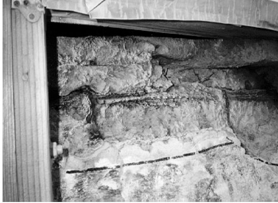
Figure 28. Close-up of the damaged concrete gallery deck after the loose concrete has been removed and before the damaged concrete was repaired using pressure-injected epoxy grout.
