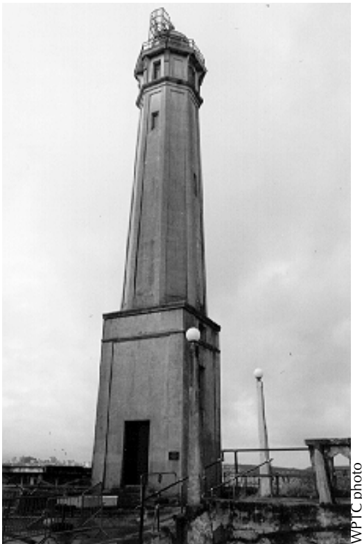
Figure 2. View of the Alcatraz Island Lighthouse. Reinforced concrete was chosen for this lighthouse location for its ability to withstand earthquakes.
