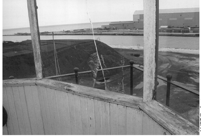
Figure 16. This lantern glass has been damaged by rock-throwing vandals. The resulting hole is allowing rain and insects to enter the lantern.
