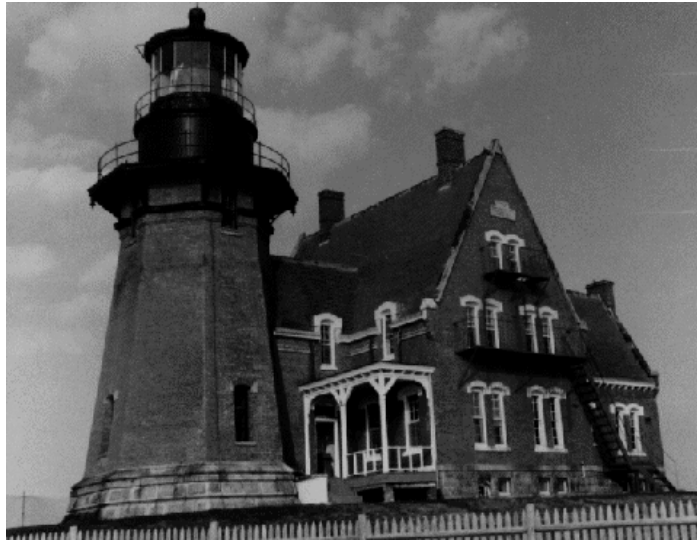
Figure 11. Block Island Southeast Light Station before the move.
