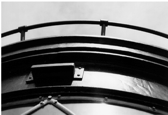
Figure 31. Close-up of the finished metal work on the lantern.
