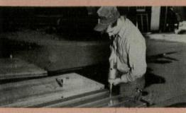
ON THE GROUND, panels are drilled for bolts which are used in erection. Two holes are positioned at the top and two at the bottom of each panel.
