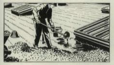
The famous Barrett Armored Surface of a triple-thick coating of pitch plus a top layer of gravel or slag assures extra protection against mechanical damage and fire.
