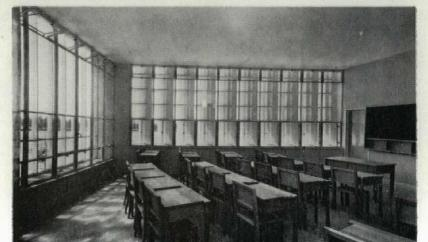
Here, adjustable vertical louvers of hollow, insulation-filled metal are ganged together and manually operated to admit solar heat on winter mornings. During hot months (which in that latitude constitute nine months of the year) the louvers are closed and the insulated fins help keep out heat.
