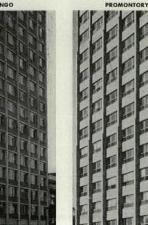
architects the local Producers' Council award for "the most imaginative and appropriate use of building materials.") The Flamingo's remarkable economy rests on a further simplification of Promontory's already simple concrete structure, plus several other cost-cutting details. (Its 75¢ cost per cu. ft\* is well below the 82-90 cent going rate for such buildings but *some* of the details represent a lower standard.)
