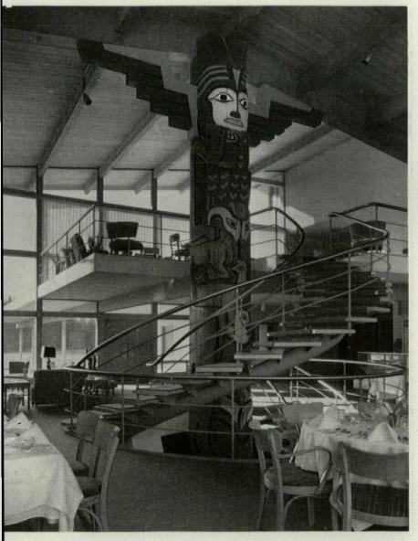
Stairway around structural totem pole is self-supporting on a formed spine of 8" steel pipe. Open carpeted treads of  $1\frac{1}{2}$ " plywood are bolted to steel angle supports welded to the pipe.
