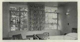
Architect Shirley Simons used Thermopane in Daylight Walls of the Smith County Hospital, Tyler, Texas, for noise and temperature control. The wall-to-wall and sill-to-ceiling use of clear glass makes the room feel less confining.
