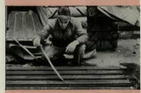
**PROTECTIVE PAPER** covering that kept the panels completely damage-free during fabrication and shipment is removed with a commercial preparation.
