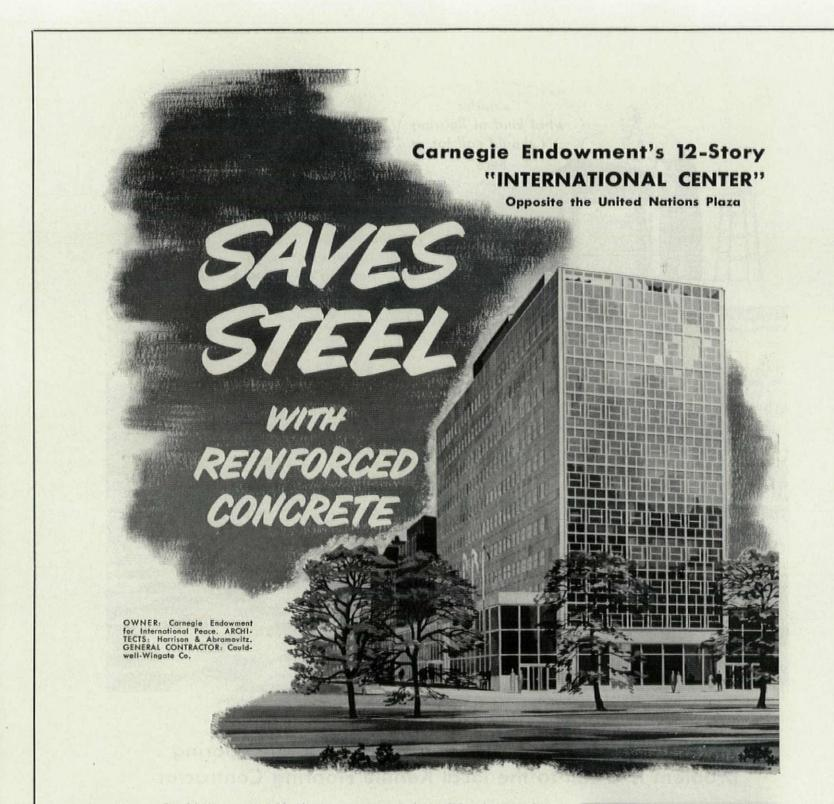
In this impressive Manhattan structure, planned for the use of nonprofit organizations active in promoting international understanding, reinforced concrete was chosen for framing and floors ... in order to *save steel* for national defense.
