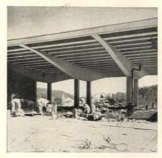
Above: The all-concrete roof covers two rows of outside classrooms and a central corridor. With its overhang, the roof is 68 ft. wide. Below: 29-ft. concrete cantilever beams extend from corridor columns over the classrooms and exterior walls.
