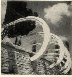
subtle but important elements of the design. The frames are about 16' long in plan and, like many other parts of the project, were prefabbed in a central casting yard.
