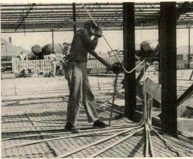
Republic "Inch-Marked" E.M.T. is approved by the National Electrical Code for concealed, exposed and concrete installations. It also meets standards of Underwriters' Laboratories and carries their inspection seal.
