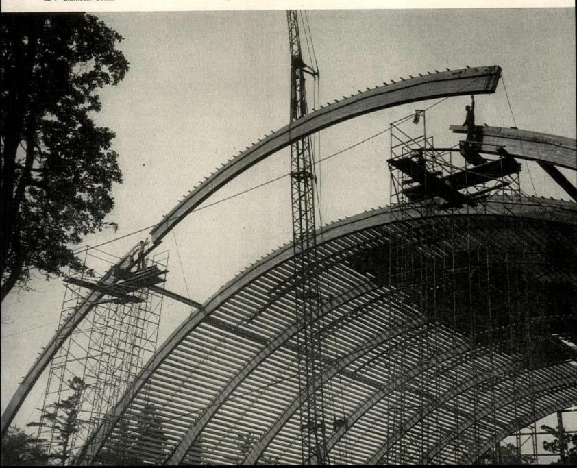
Union College field house uses 247' frames to cover 190'; Montana's uses flatter 226' arches to span record 201'
