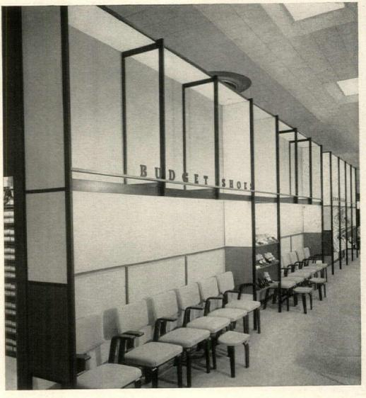
ONE-WAY FIXTURES are backed by stock cabinets to form storage-display partitions. Photos show design variations to accommodate shoe-fitting chairs, sporting goods and glassware. Note wide variety of materials used with standard hollow metal framework.
