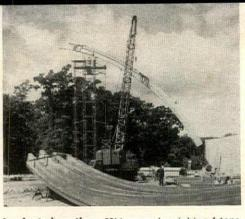
Laminated section, 83' long and weighing 4 tons, is raised between hinge and erection tower. Left, detail of splice.
