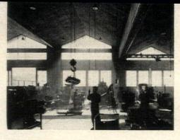
**Shop interior** of 36'-wide bays is roofed with 6"-thick folded slabs tied by precast beams at ends. Roof carries 15-ton cranes.
