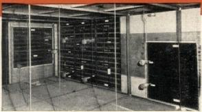
Inside this duct Johnson Damper Operators and Dampers insure precision control of the minimum and maximum outdoor air supply for Weathermaster units throughout the building.
