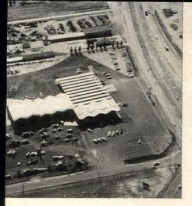
Air view of equipment factory shows shop area on left, with 36' x 80' folded plate slabs, a display area in front with 40' x 80' folded slabs cantilevered 28' forward of supports, and an office and parts area in rear with Z-shaped northlight slabs.
