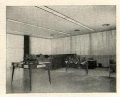
A noise-absorbing ceiling of Travertone prevents reflecting sounds from hard-surfaced walls and floors in the main banking area from creating a serious noise problem. The resulting quiet atmosphere lends dignity to the bank's modern design.
