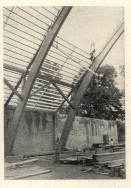
**K-trusses** of laminated timbers up to  $9'' \times 24''$  in section span 25' between arches.
