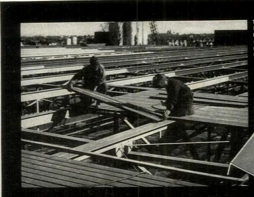
Time is money on every building job. Milcor Steel Roof Deck gets operations under cover fast at low labor cost, gives ideal base for permanent roofs.
