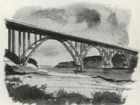
CANIMAR RIVER BRIDGE, CUBA CONSTRUCTED BY RAYMOND
