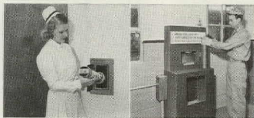
Left: Nurse inserts carrier. System handles test tubes, charts and other hospital items. Right: Pneumatic tube station in laboratory office of steel mill.
