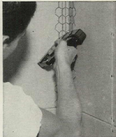
Use either nails or staples with Keycorner. For use over doors or windows, or as strip lath, it can be pressed flat to provide a smooth surface for plastering.
