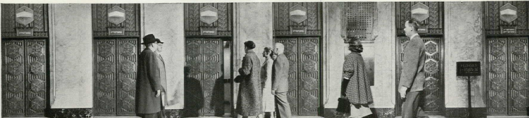
Elevator doors open automatically as car arrives
