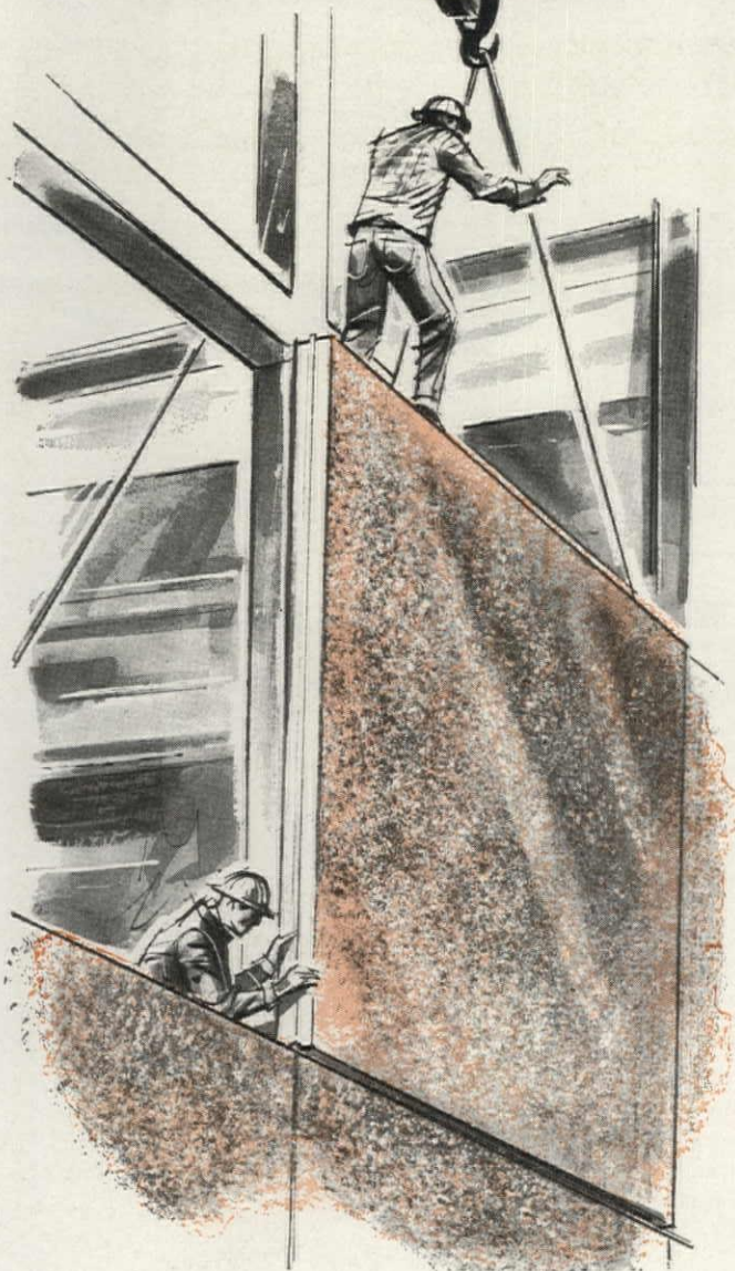
The new Goodyear Research and Development Center at Akron, Ohio, features the use of Marietta panels with lift-slab construction.
