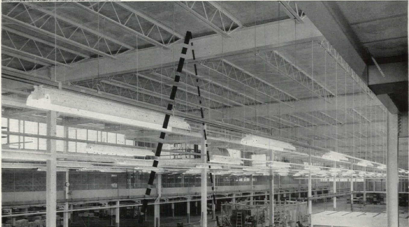
Building: National Lock Co., Rockford, Ill. Architect: Ragnor-Benson, Inc.
