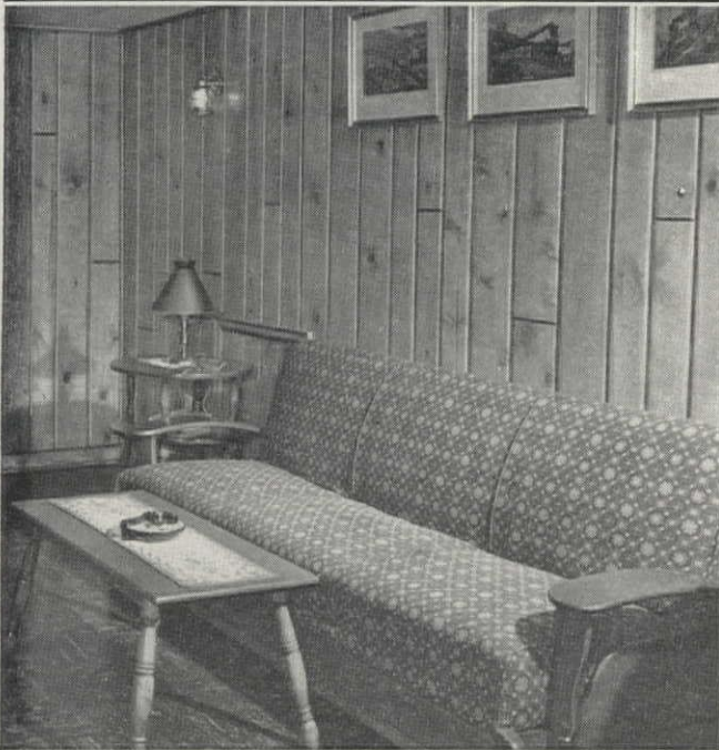
NU-WALL: Ponderosa Pine paneling with random Vee horizontal end-matching. Kiln-dried and packaged to specified 7' or 8' lengths. Comes in three distinctive stylings: Formal (clear), Traditional (small to medium knots) or Contemporary (medium to large knots).
