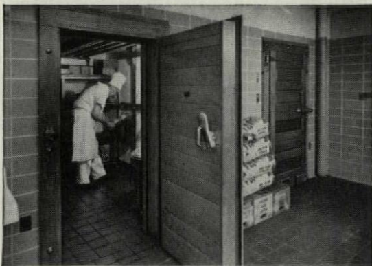
Both walk-in refrigerators are insulated with Styrofoam.
