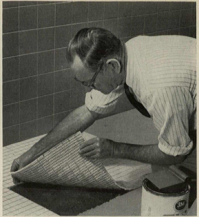
With Perma-Bak, the tile setter can see what he is doing. Chance of error is greatly reduced.
