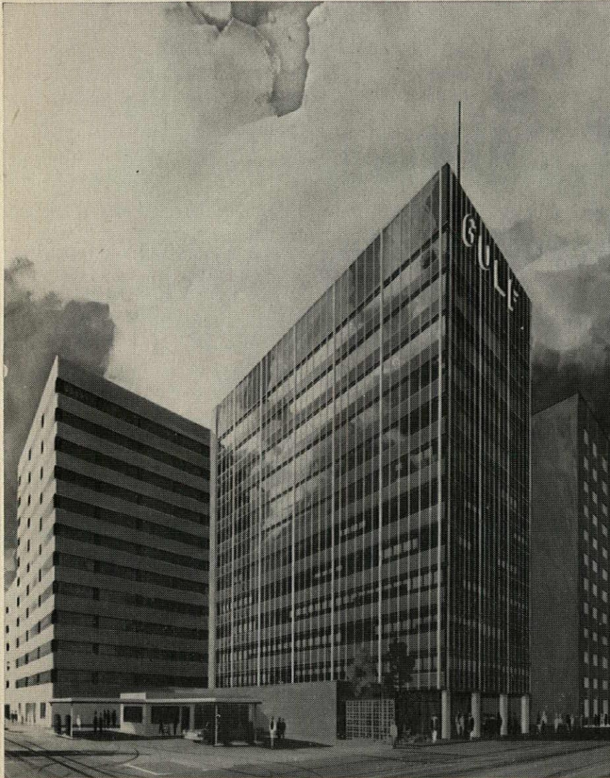
GULF BUILDING—Midland, Texas. Owner: R. E. Dumas Milner, Jackson, Miss. Architects: Hedrick and Stanley, Fort Worth, Texas. Plumbing Contractor: Davis Plumbing Co., Jackson, Miss. Plumbing Distributor: Paine Supply Co., Gulfport, Miss.
