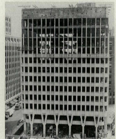
Double-duct high-velocity air conditioning , as used in the Blue Cross-Blue Shield Building, delivers both hot and cold air to each room where it can be mixed in any proportion to supply either heating or cooling as required.
