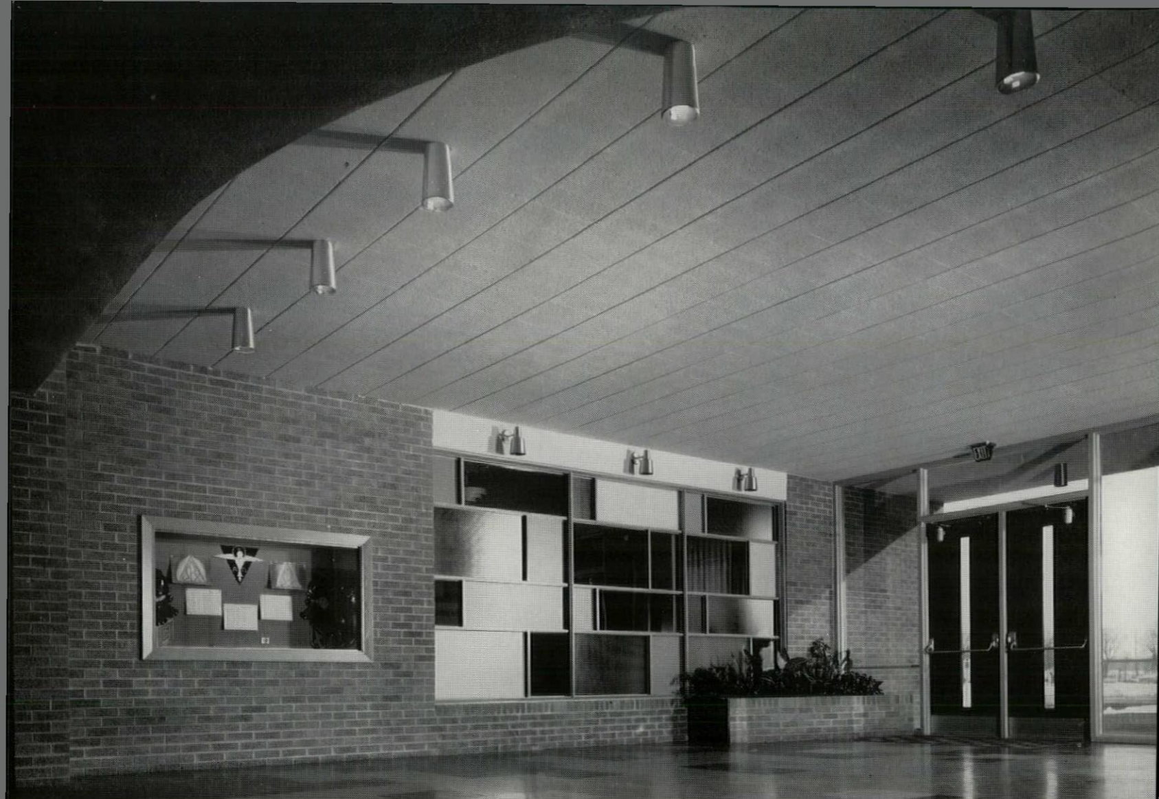
Flush block ceiling blends well with other masonry. Long unbroken spans.
