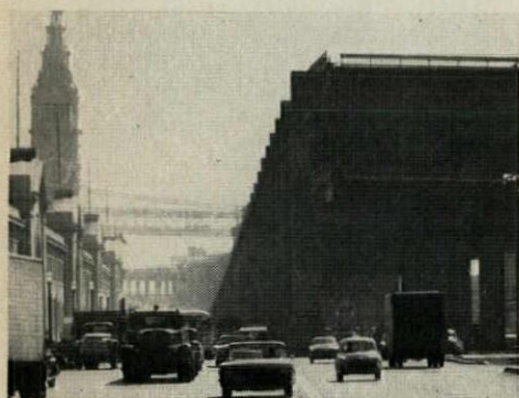
"A double-deck expressway down the Embarcadero, ruthlessly cutting in front of the Old Ferry Terminal, robbing the water front of sunlight and bay view."
