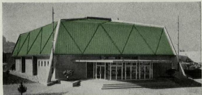
Memorial Building of the International Longshoremen's and Warehousemen's Union, San Francisco. ARCHITECT: Henry Hill, San Francisco. The dome is sheathed with about 18,000 sq. ft. of Economy Copper Roofing installed by Fire Protection Products Co., San Francisco.
