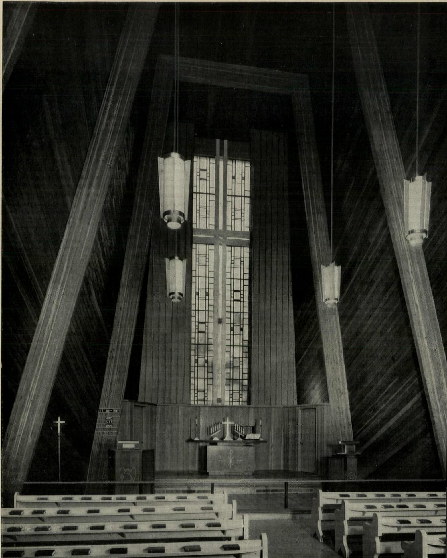
Allowing wood to function structurally and decoratively helped realize significant economies in the construction of this modern church. These dramatic supporting members are 2x6's over laminated arches. Sargent, Webster, Crenshaw and Folley, architects.
