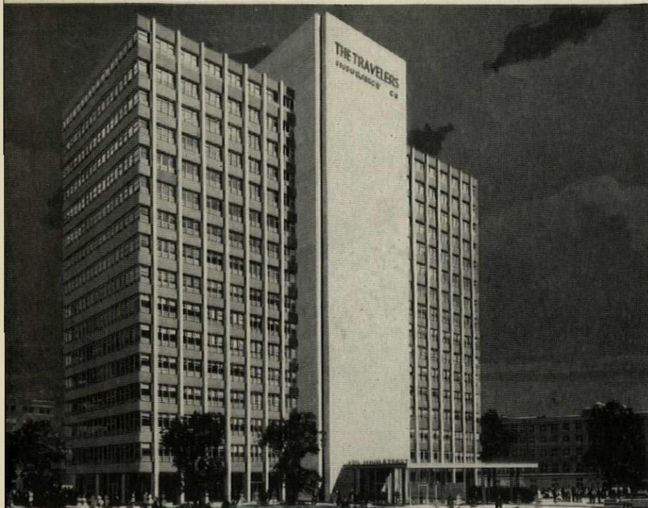
Sprinkler System and Stand-Pipe Fire Lines in Travelers Insurance Boston building are durable steel pipe. Savings in initial and installation costs were considerable; insurance premiums were less with steel pipe fire protection systems on guard throughout the structure.
