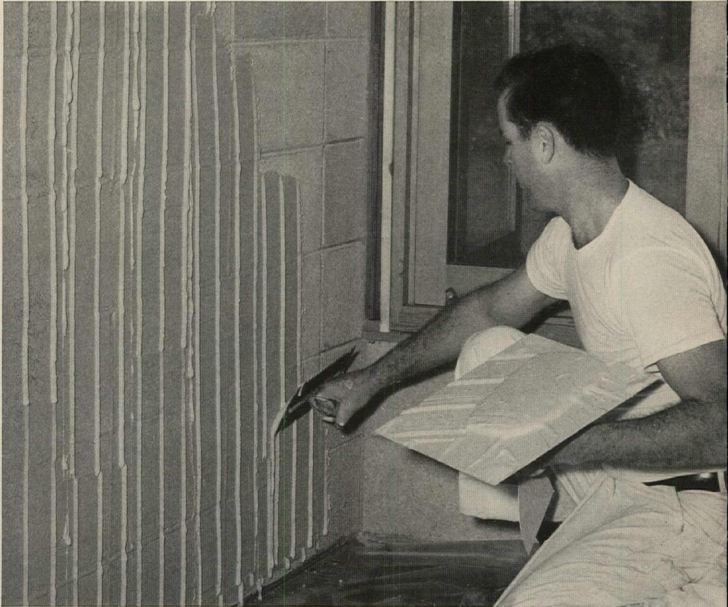
After Styrotac™ bonding cement is applied to either the wall or to Styrofoam, the insulation is pressed in place (center). After overnight setting, gypsum wallboard is either spot-coated or notch-trowelled with Styrotac and pressed in place over the Styrofoam insulation (right).
