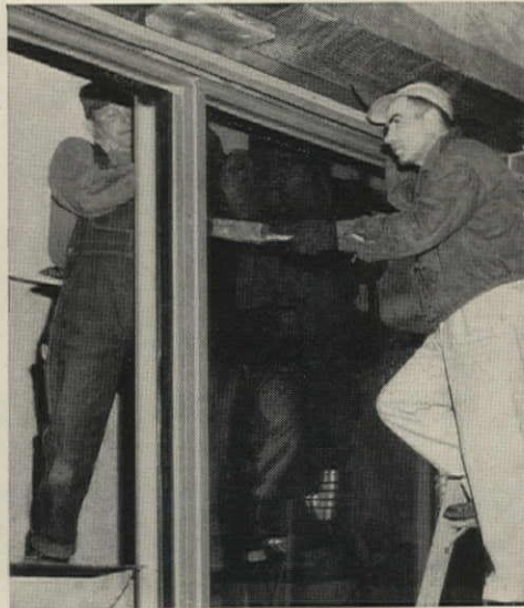
3. Glass unit is worked into gasket with special tool.
