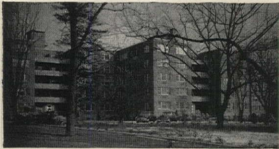
Trouble-free Donley Incinerators were specified for this large residential development in Philadelphia.
