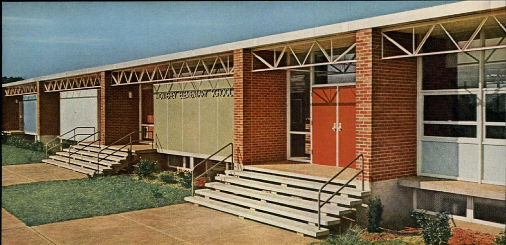
Design conditions in Monterey Elementary School, Roanoke, Va., required the use of two types of Glasweld panel—relatively small insulated sandwich units finished both sides and large uninsulated panels. See detail below right. Architects: Frantz & Addkison-Caudill, Rowlett & Scott, Roanoke, Va.
