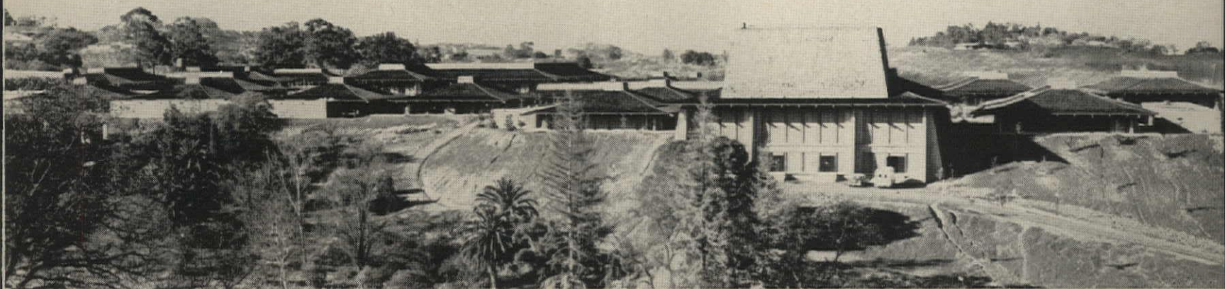
Auditorium rises along the campus' south side. Plans below show how the "space module" is multiplied, combined with office and lecture units.
