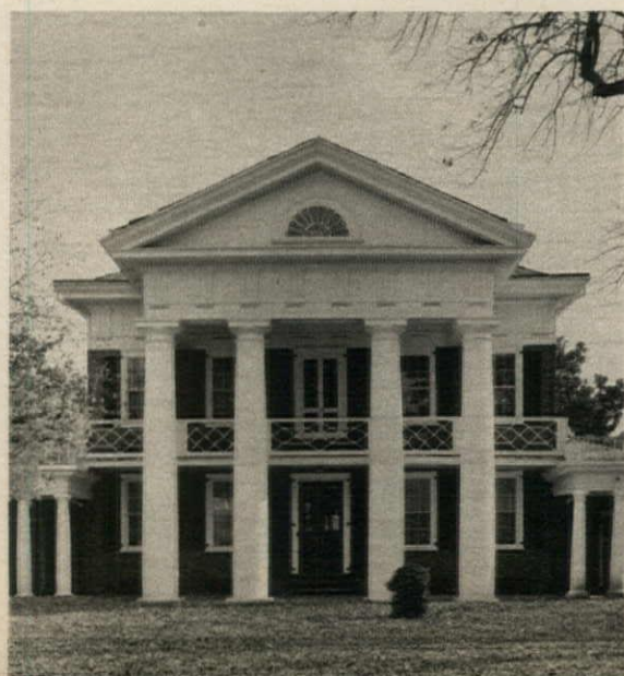
Note how colonnade and balcony join in Pavilion X.
