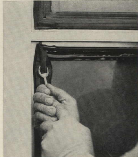
4. Neoprene strip, "zipped" into gasket, serves as locking device.
