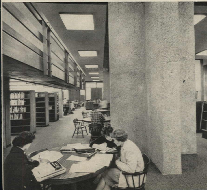
Typical massive piers of pebbled concrete rise here in the library. Space under hipped roofs is revealed only in octagonal lecture halls.
