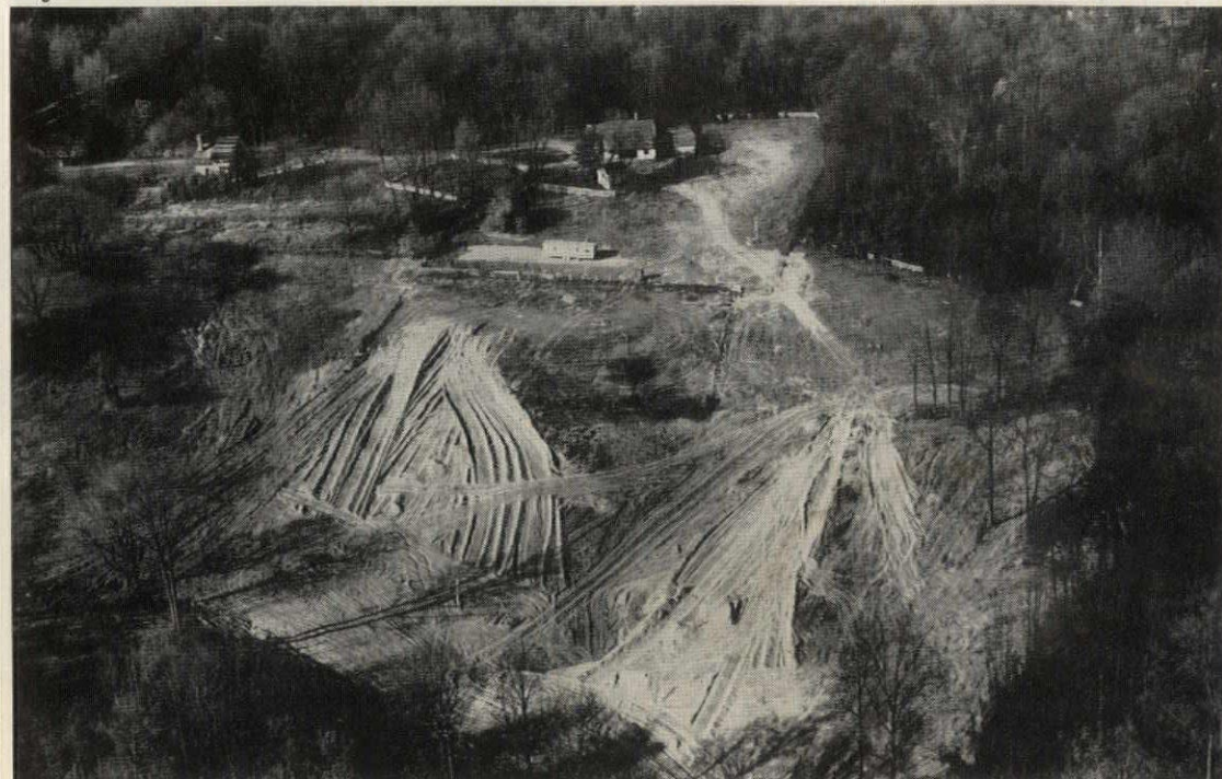
Magazine Brothers' excavation at Potomac Palisades
