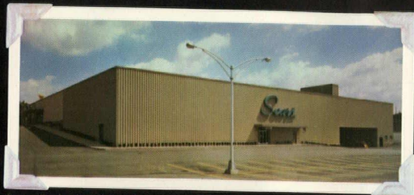
Sears, Roebuck and Co., Greensburg, Pa. Architects; Kuhn, Newcomer & Valen- tour, Pittsburgh. General Contractor; Westmoreland Construction Co., Greensburg
