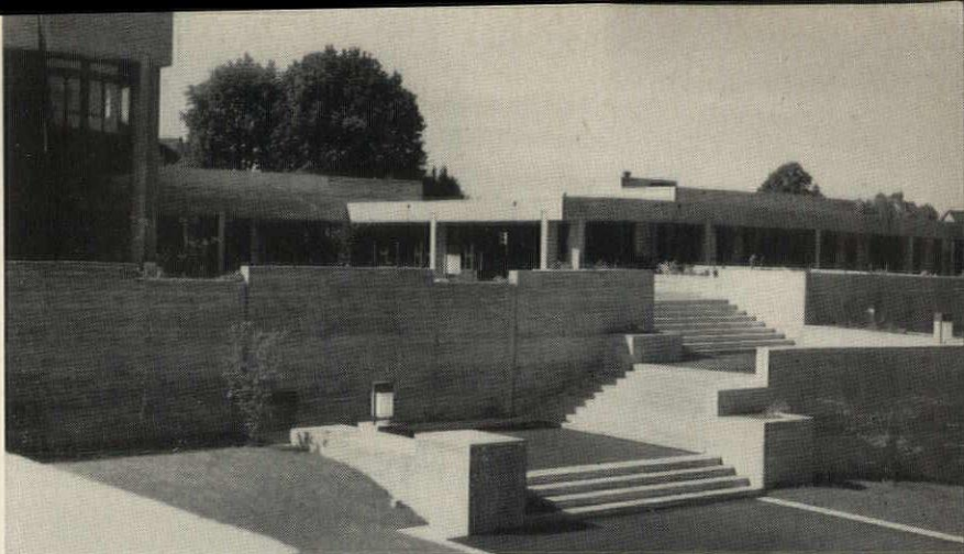
Broad steps lead up to hilltop campus located 50 feet above access road
