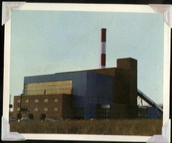
McKee Run Generating Station, City of Dover, Delaware. General Contractor; Somers Construction Co., Bala Cynwyd, Pa.
