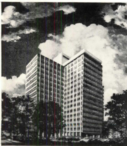
The Travelers Insurance Co., new Boston office building. Kahn and Jacobs, Architects. Jaros, Baum and Bolles, Consulting Engineers. George A. Fuller Company, General Contractors.
