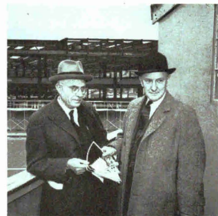
(Left) Dr. Pier Luigi Nervi, the noted Italian engineer, is shown with John M. Kyle, chief engineer of the Port of New York Authority, on a recent inspection tour of the George Washington Bridge Bus Station being built by the Port Authority. The two-block-long, three-level station, to be completed in the summer of 1962, is the first building in this country designed by Dr. Nervi
