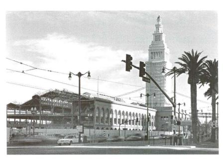
As construction proceeded, surprisingly little of the original Ferry Building fabric proved salvageable. A continuous second-floor bay was added on the water side.
