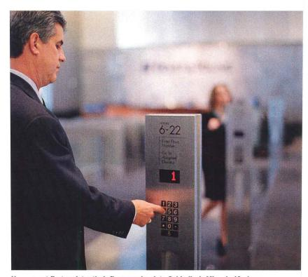
Users must first register their floor number into Schindler's Miconic 10 elevator group control system before entering the elevator.
