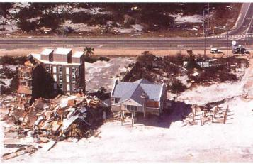
Multistory buildings are usually considered well-enough engineered to withstand a hurricane. But in Orange Beach, a medium-rise building collapsed due to undermining and direct wave attack during Hurricane Ivan.
