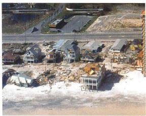
A row of houses in Orange Beach, Alabama, were inappropriately sited on top of a dune instead of behind it, leading to significant damage.
