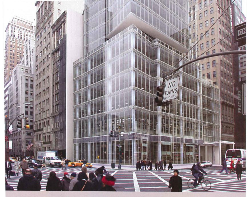
Thin concrete floor plates made it possible to get an additional two floors in the envelope. The floors are cantilevered 15 feet from the columns, which required careful detailing of the curtain wall to accommodate deflection and shrinkage.
