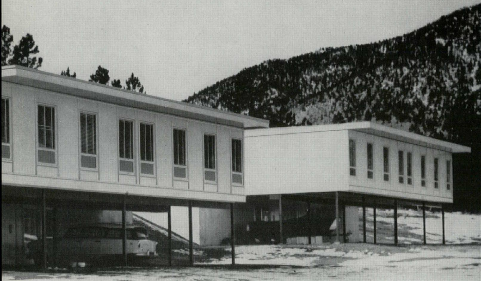
BELOW—Two Andersen Strutwall units butted together result in this handsome picture window effect. Lower operating sash are awning type. Permit ventilation even during rain storms.
