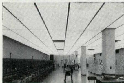
Installation of Contrex Soundsheet — Operating Room, Forest Hills Telephone Building, New York Telephone Company.
