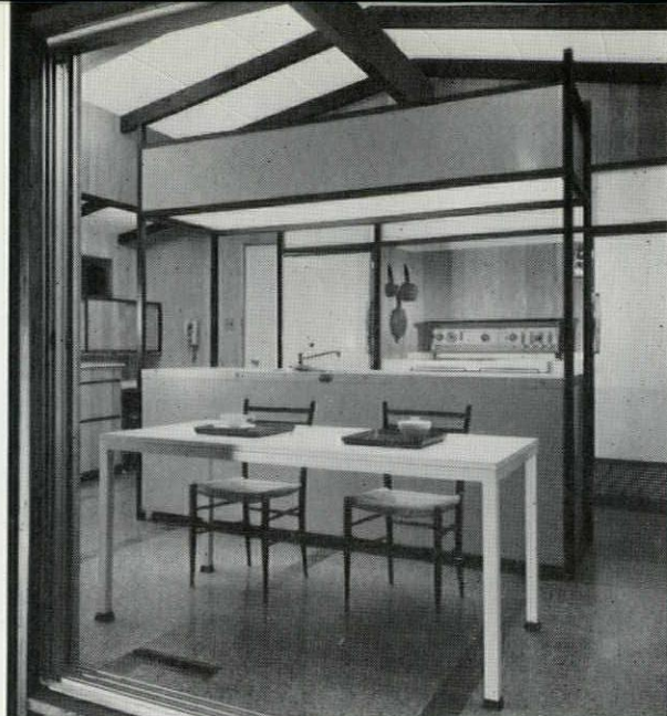
Kitchen dining area. Architect David Leavitt, AIA, is a partner in Leavitt & Henshell, New York City.
