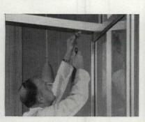
EASIER SPEED ADJUSTMENTS than with floor-check entrances. Kawneer Concealed Overhead Closer has two closing speeds, and has independent adjustments for both closing speed and latching speed. Also equipped with spring tension adjustment for severe wind conditions, independent of the hydraulic action of the other two speeds.
