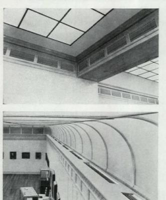
The photograph above illustrates an Anemostat Straightline Air Diffuser installation in the gallery design of the Sterling and Francine Clark Art Institute at Williamstown, Mass. The conditioned air is supplied through Straightline Diffusers located on all four sides of the gallery. The diffusers not only draftlessly introduce conditioned air into the gallery, but also blend into the architectural design.
