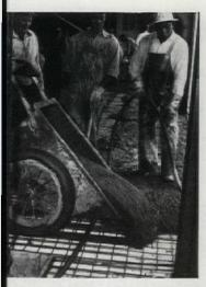
RANCO PRODUCTS PROVIDE RM BASE for concrete. Unobacted work area speeds concreting, wood forms. No wasted fill. Reinced concrete construction. Granco ducts are available in a number of this and gages to help you meet ious load conditions.
