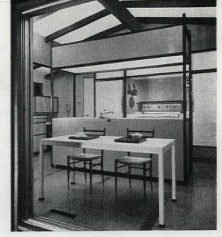
Home is designed on 3' module with four roof heights. Highest is over the living room,
