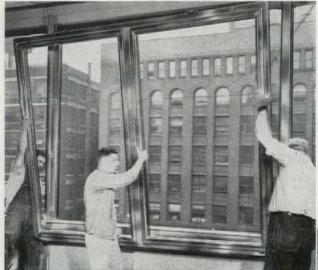
STAINLESS STEEL REVERSIBLE WINDOWS, here being installed, and Stainless Steel Curtain Wall, used throughout the new Morton Salt Company Office Building, were fabricated by Republic's Truscon Division. Architects: Graham, Anderson, Probst & White, Inc., of Chicago, Illinois. Contractor: Sherman Olson, Inc., also of Chicago.
