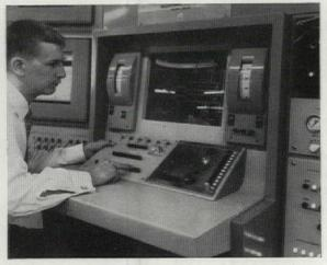
Figure 9—Two pushbutton consoles similar to one shown (below) will control 60 floors of new Chase Manhattan Bank Building, New York. Diagrams of heating and airconditioning systems for each floor can be projected on screen.
