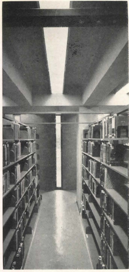
The structure is based on a 5-ft stack module: stacks are directly over concrete beams 5-ft o.c., which are left exposed at the ceiling to form troffers for continuous lighting.
