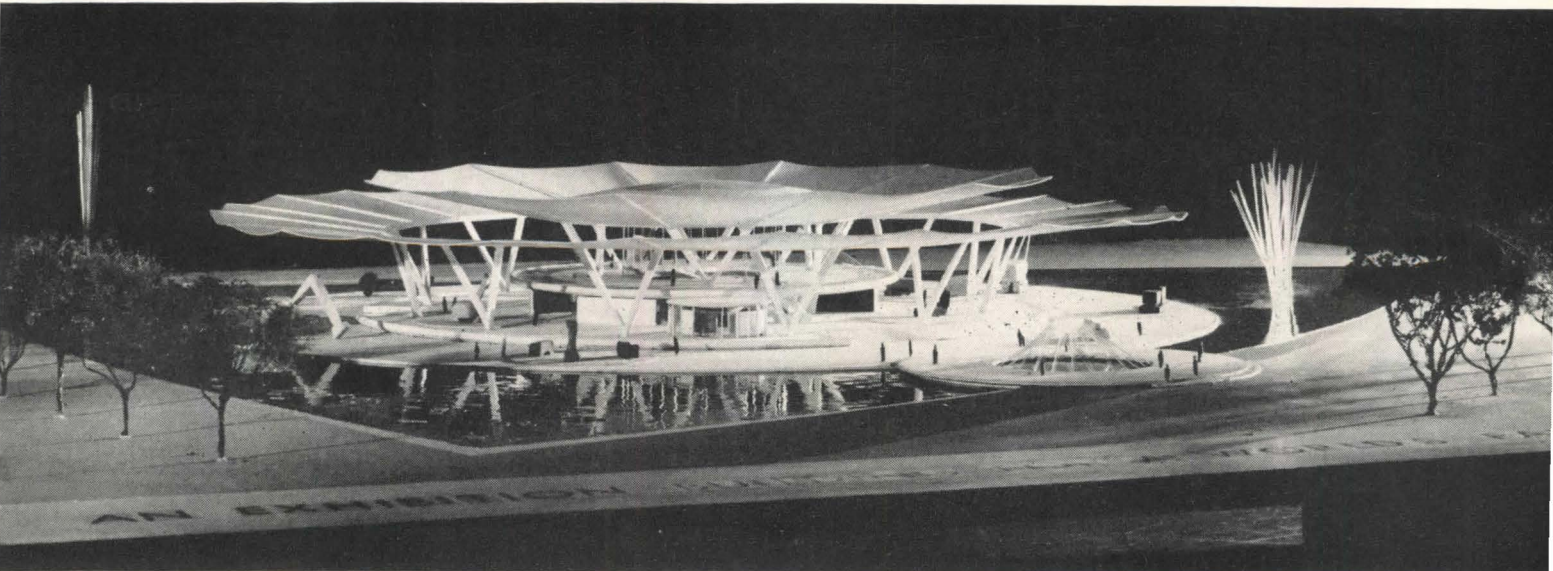
Axially-stressed strut-and-column system, carrying concrete membrane between struts, covers 126,000 sq ft of usable area at ground level.
