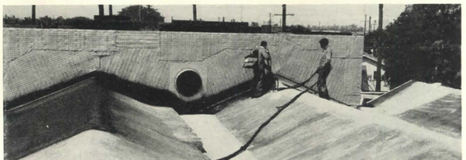
Flexibility of Monoform permits use on many shapes of roofs.
