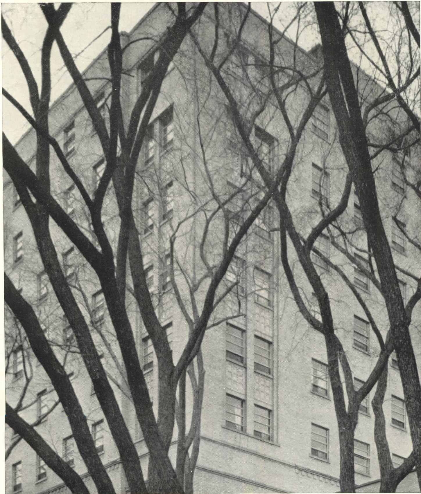
MILLARD FILLMORE HOSPITAL, Buffalo, N. Y. Architects: Kidd and Kidd.
