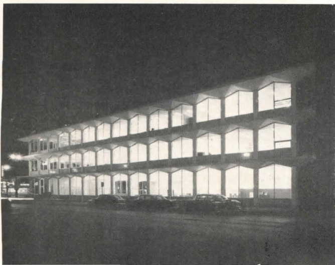
The number of columns has been doubled along the façade to create a strong rhythmic pattern which is emphasized by night lighting.
