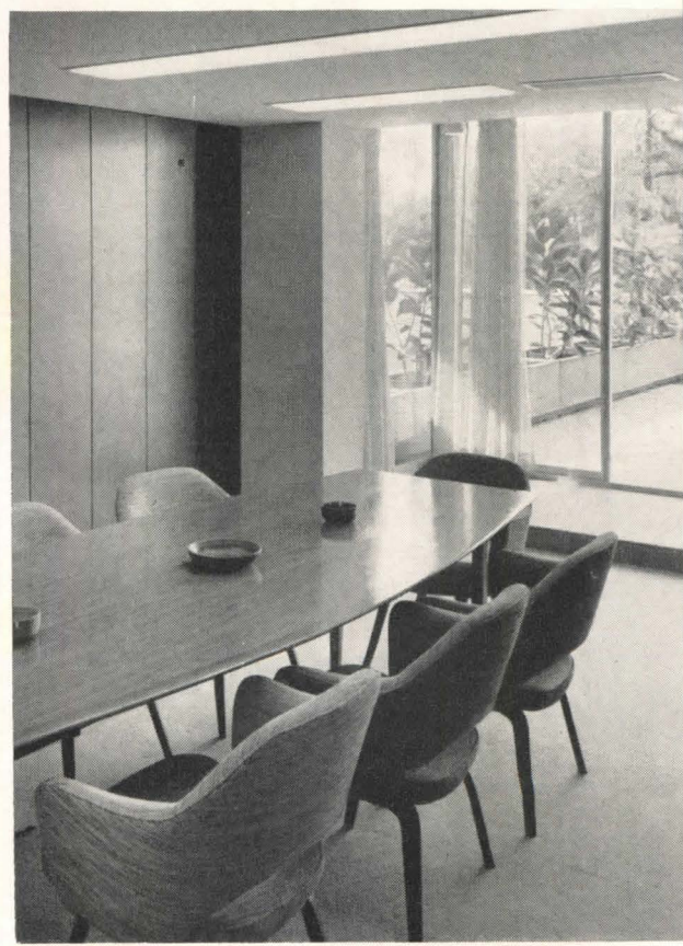
The structure is based on a 5-ft stack module: stacks are directly over concrete beams 5-ft o.c., which are left exposed at the ceiling to form troffers for continuous lighting.
