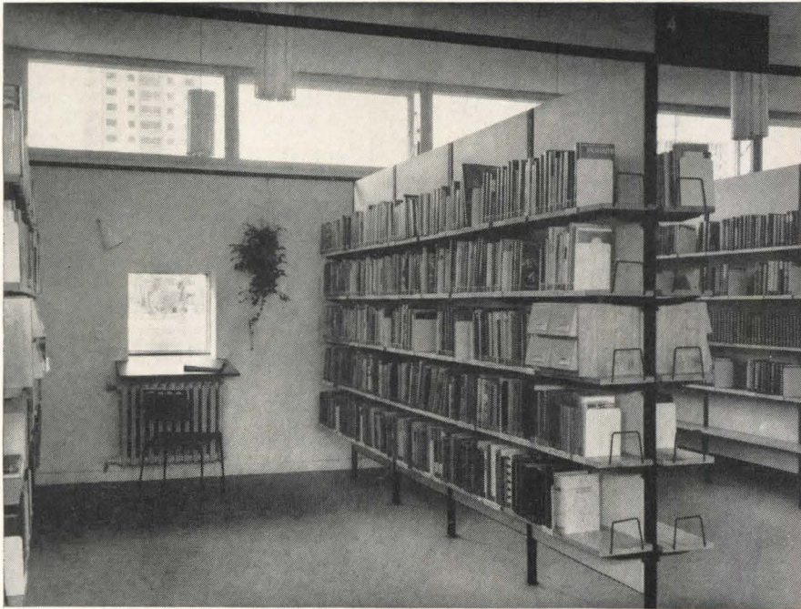
The reading room (top), has window walls on both sides; informal, light furniture may be moved into the garden. Plaster ceilings around the outer part of the library are higher than the wood ceilings. Freestanding book stacks are supported on metal uprights with adjustable brackets carrying wood shelves; they, as well as the display cases and book carts, were designed by the architect.
