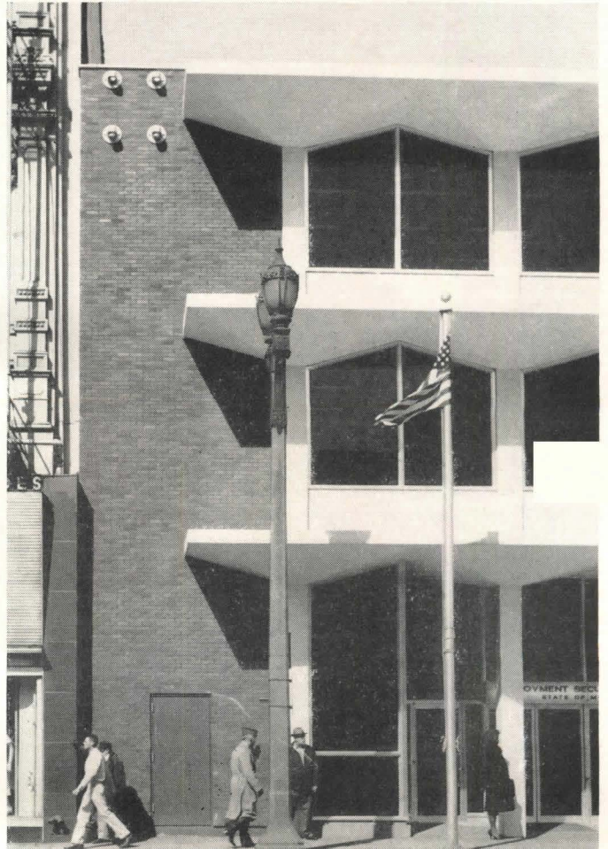
The inverted-pyramid structural forms of the St. Louis building are carried out beyond the glass to form a continuous colonnade.
