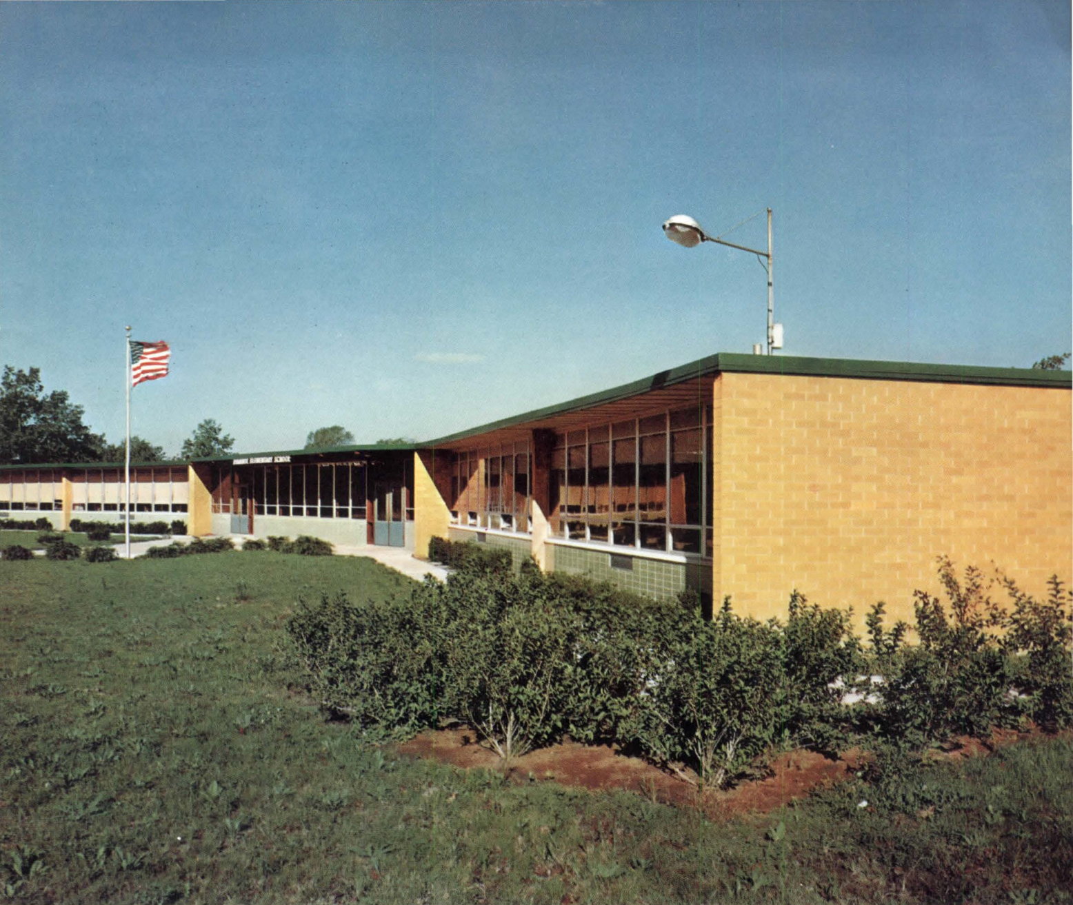
View of the modern Ivanhoe Elementary School in Gary, Indiana, showing its walls of Natco Uniwall. The buff colored vertical walls show Uniwall's exterior rugg-tex finish. The light green panels under windows show a unique use of Uniwall's interior face installed in reverse. Architect: Jos. P. Martin & Assoc.
