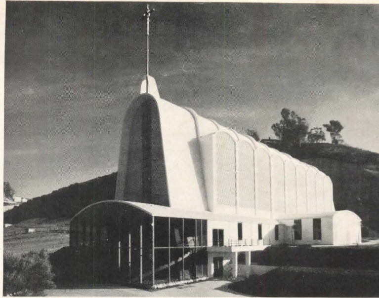
(Above) First Methodist Church, San Diego, California. Architects: Perkins & Will. Structural Engineers: Rutherford-Chekene. General Contractor: M. H. Golden Construction Co. Prestressed Elements: San Diego Prestressed Concrete Co. Pozzolith Ready-Mixed Concrete: San Diego Consolidated Rock Products.
