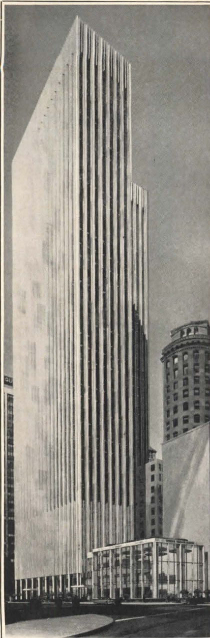
Wells Fargo Building, San Francisco, tallest building west of Dallas. Owner: Dillingham Corp. Honolulu, San Francisco. Architect and Engineer: John Graham and Company, Seattle and New York. Plumbing Contractor: Scott Co., Oakland, California.
