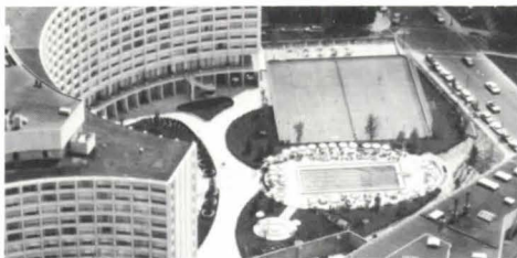
Roof-top and Other Above-ground Installations
