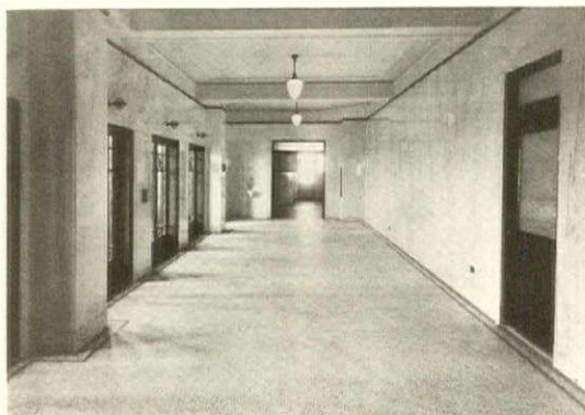
A typical upper corridor in the Jefferson Building, showing use of Alabama Cream A marble
