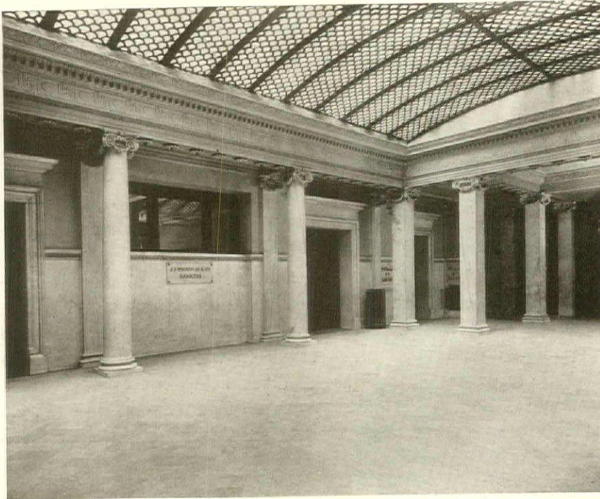
Lobby of the Calvert Building. These marbles successfully withstood the Baltimore fire.
