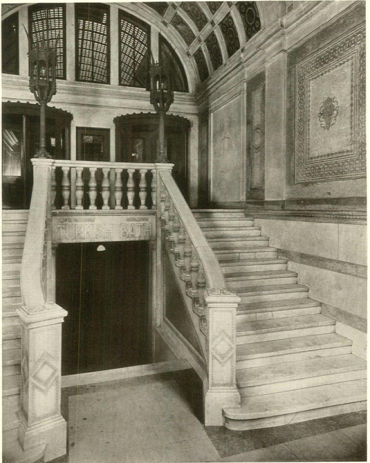
Entrance to the Equitable Building, Baltimore, Maryland. These marbles came unscathed through the fire of 1904, that leveled hundreds of buildings built of brick and other materials.
