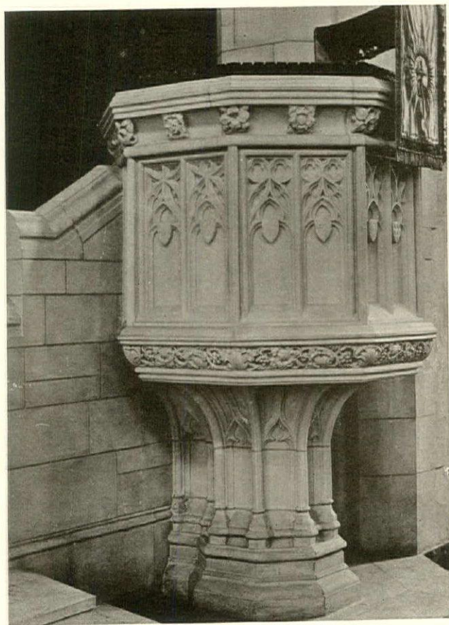
Pulpit of the Second Congregational Church at Holyoke, Massachusetts, executed in English Bath Stone.
