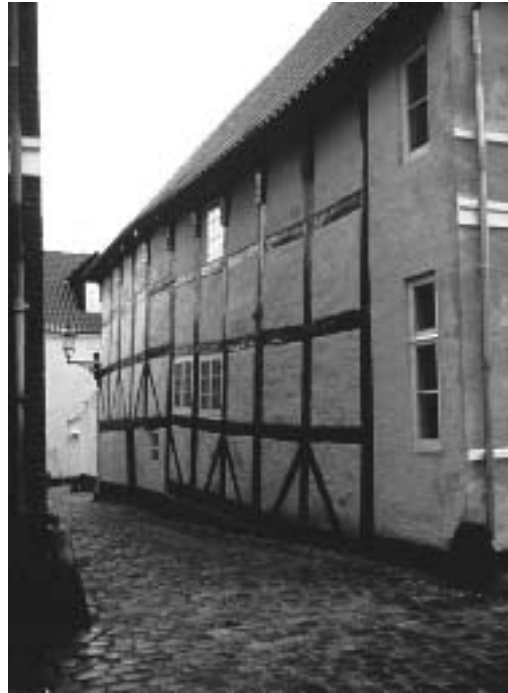
Fig. 4.3: This house in Grønnegade in the city of Ribe dates back from around 1530. It is a good example of the timber-framed houses from the 1500s. The façade was brick-built in 1848, which is also a typical feature in the development of the timber-framed townhouses. Photo: S. Søndergaard
