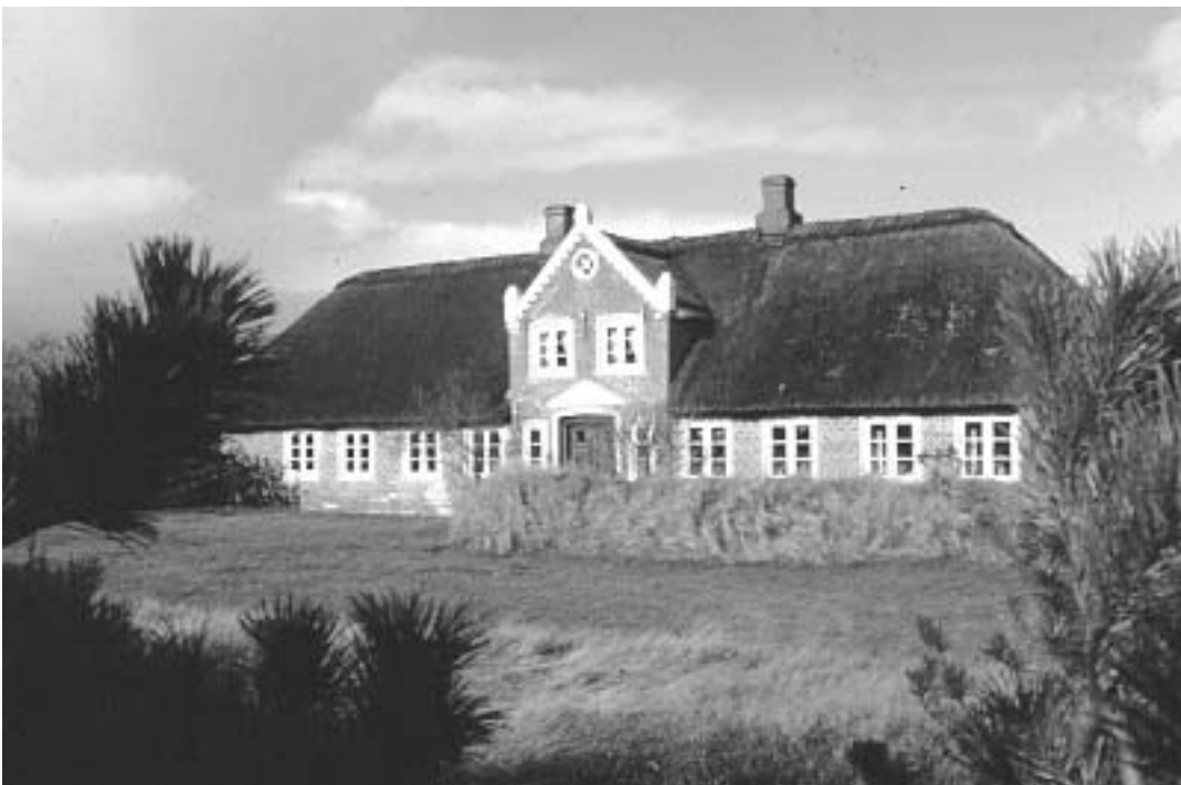
Fig. 2.9: Farmhouse in the Ballum marsh, Denmark Photo: J. Frederiksen
