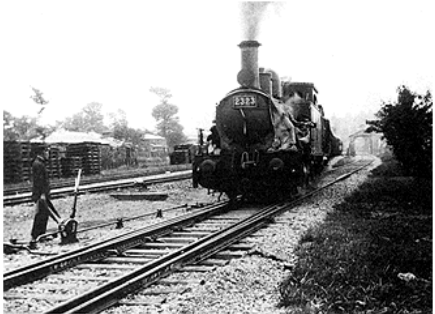
■ Mixed-Gauge Test Track near Tokyo
