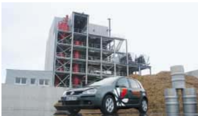
The first stage of the new plant was commissioned in October 2003
