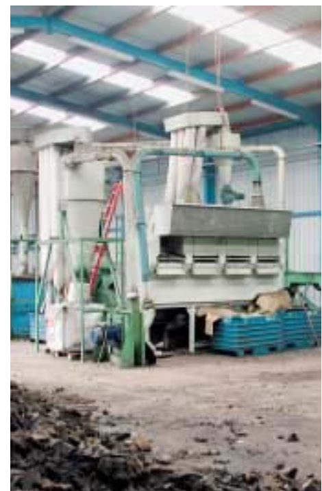
Equipment for processing shredder residues
