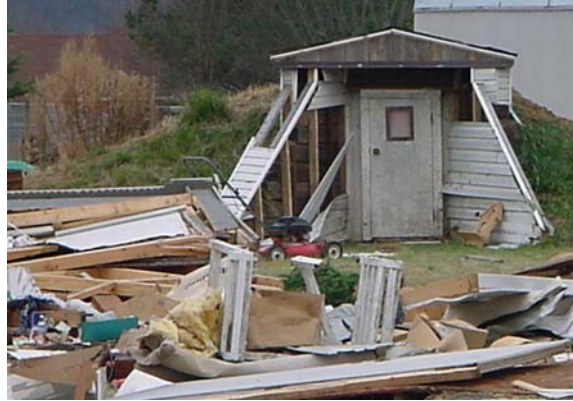
An F2 tornado struck New Hope (Madison Co.) on November 24, 2001. This storm shelter remained completely intact while the house nearby was destroyed.
