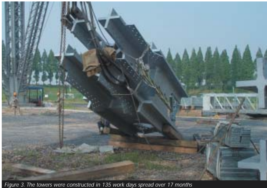
Figure 3. The towers were constructed in 135 work days spread over 17 months
