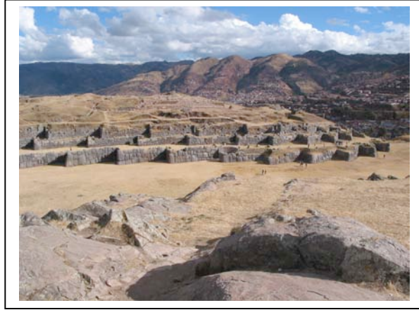
Looking towards Baluarte where the zigzag wall is located from the mullion.
