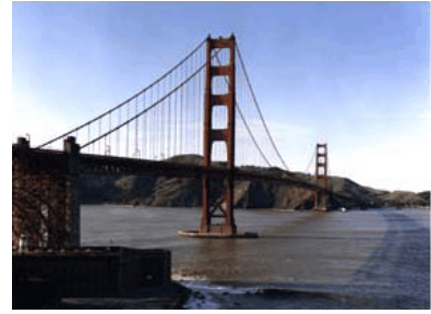
GOLDEN GATE BRIDGE
