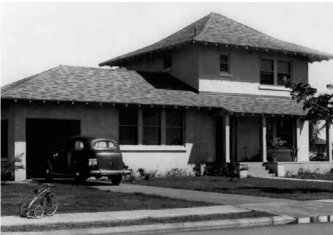
Officers' House plan "J" (Quarters 544) at Hickam Air Force Base as it appeared newly constructed in 1938. (Source: Mason Architects, Inc.)
