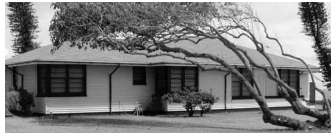
Front view, Senior Officer's Quarters (Facility 512) at the Marine Corps Base Hawaii. Constructed in 1941. (Source: Mason Architects, Inc.)
