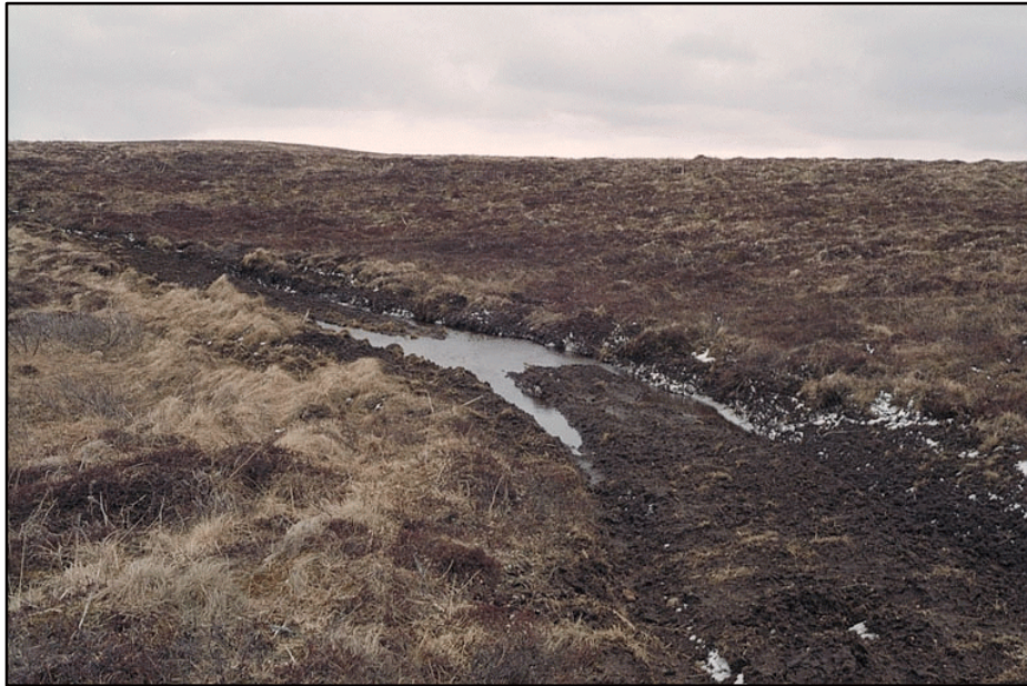
Figure 2a. Water-filled ruts on the Outpost Road, Izembek National Wildlife Refuge.
