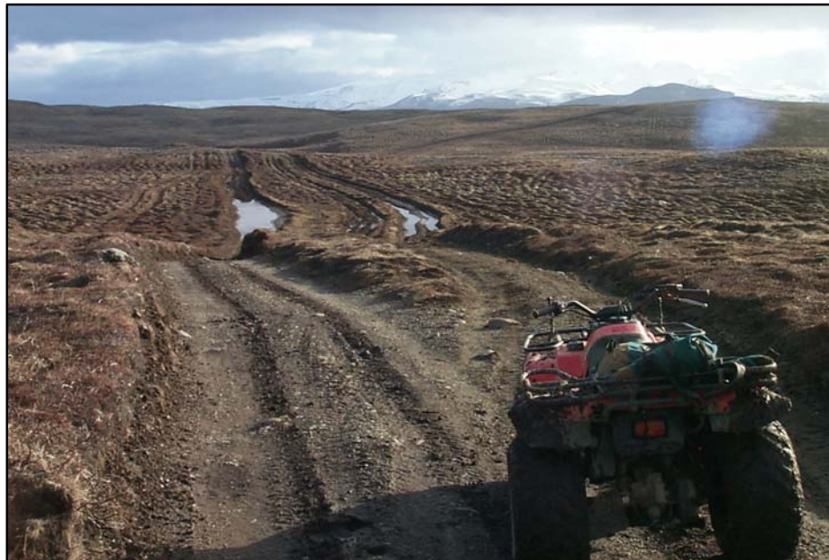
Figure 2b. Braiding of road to avoid water-filled ruts on the Outpost Road, Izembek National Wildlife Refuge.
