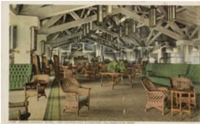
Lounge facing toward the staircase and lobby.
