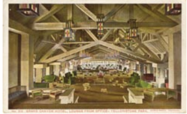
Lounge from the lobby at the top of the staircase.
