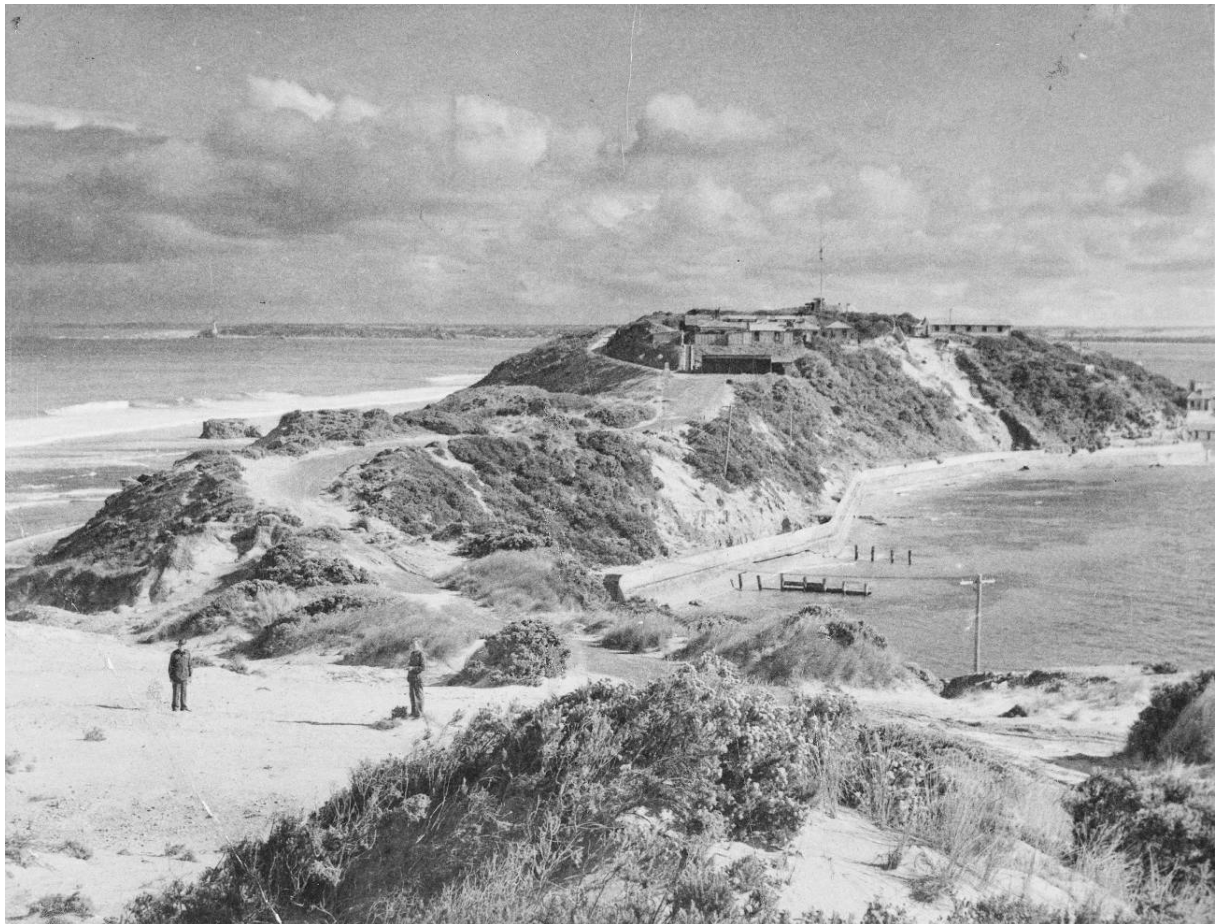
Fig. 6. Looking west to Fort Nepean, c.1946. Barracks blocks and other ancilliary timber buildings are visible, now demolished. As well, sea walls constructed to retard erosion of the Point are clearly apparent. (Australian War Memorial, Canberra, ID PO1108.011)
