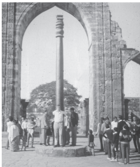
Figure 4. The ancient Delhi Pillar, made by forge-welding pieces of wrought iron. Its surface is remarkably free of corrosion.
