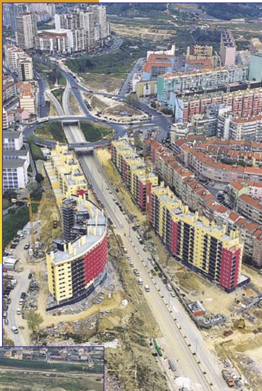
JARDINS EXPO – Construção dos Lotes RTB6 e RQ3 nas Olaias, Lisboa – Construction of Housing Buildings, Lots RTB6 and RQ3 at Olaias, in Lisbon
