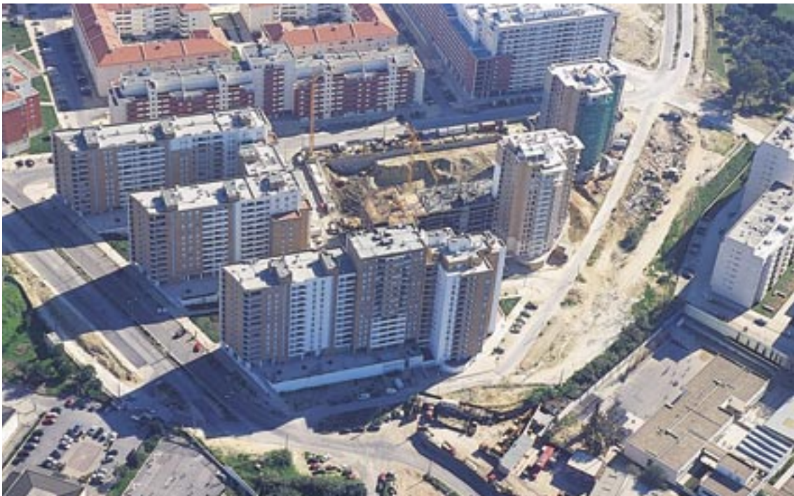
□ SGAL – Construção dos lotes 3.9/3.10 – Lumiar, Lisboa – Construction of Lots 3.9/3.10, Lisbon
