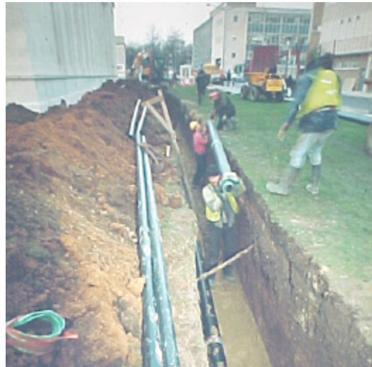
Picture 1. Mains being laid alongside the Civic Centre
