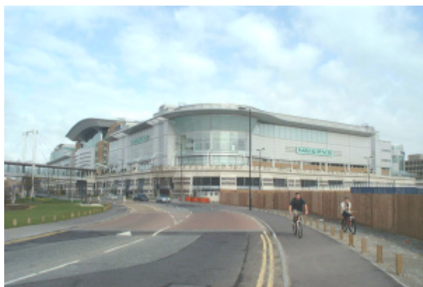
Picture 3. The West Quay shopping centre under development
