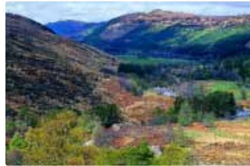
Cuileig Power Station viewed from above
