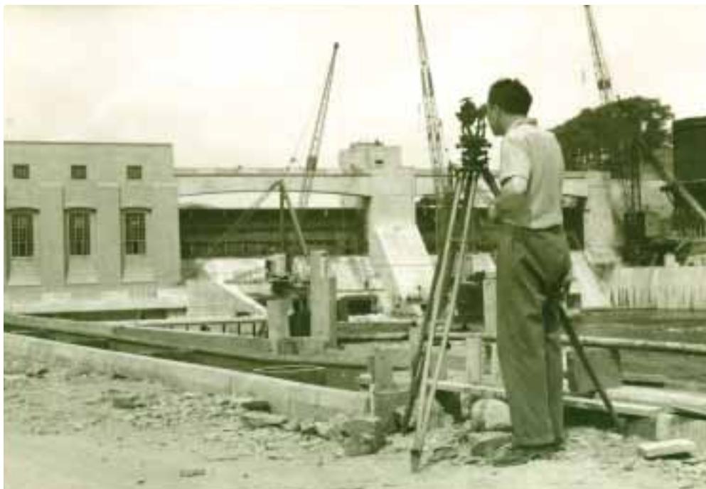
Surveying during construction at Pitlochry
