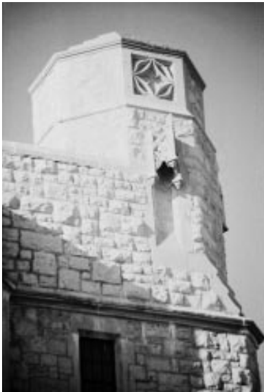
A tower element such as that on Holden Hall could define the east end of the Rampart buildings.
