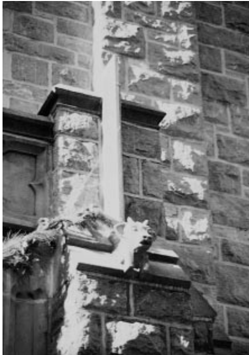
Traditional carved stone figurative ornament. Reflecting the craft of its time, it embellishes a functional rain shedding cap along a buttress.
