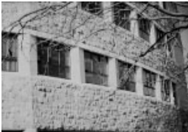
Contemporary hokie stone wall with openings trimmed in finished limestone
