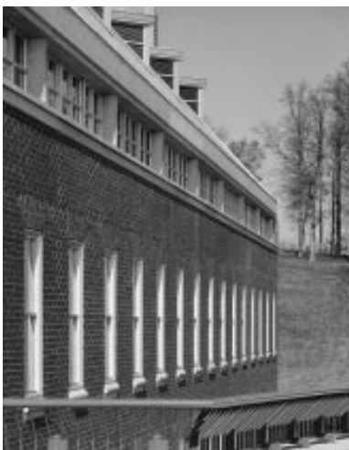
Profiled aluminum extrusions allow economical and maintainable modern windows of a traditional nature. George Washington University, Loudoun County, Virginia.
