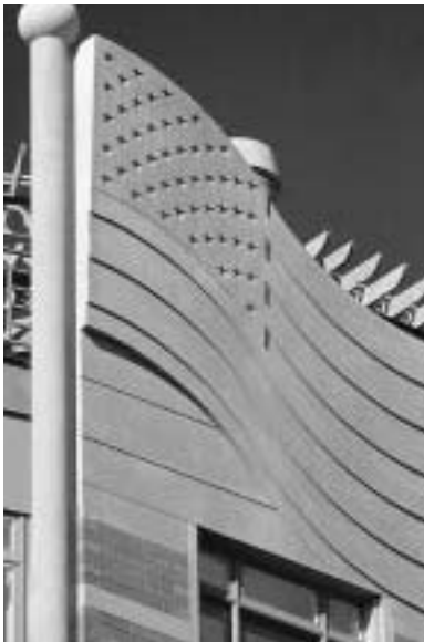
Contemporary ornament and detail achieved with cast stone on an office building. Pennsylvania Avenue, Washington, D.C.
