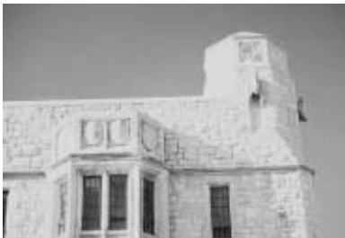
Roofline features, Holden Hall
