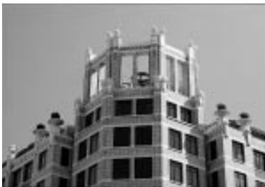
Cast stone and patterned brick are economical means for producing contemporary roof line ornament. Republic Place, Washington, D.C.
