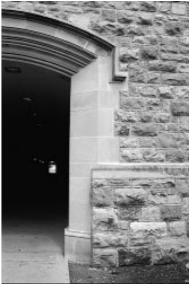
Traditional stone detailing organizes the effects of weathering to enhance architectural expression.
