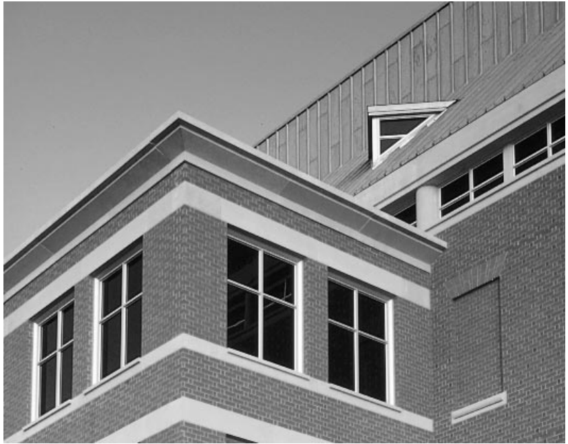
Contemporary example of architectural detailing achieved with cast stone. George Washington University, Loudoun County, Virginia.
