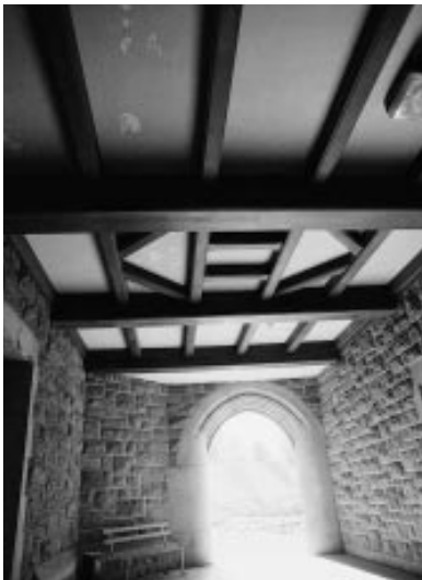
Passageways are finished, exterior vestibules.
