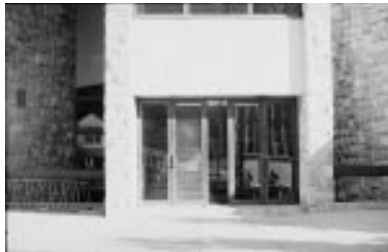
The entry and doors above are not compatible with Virginia Tech's architectural tradition in style or quality.
