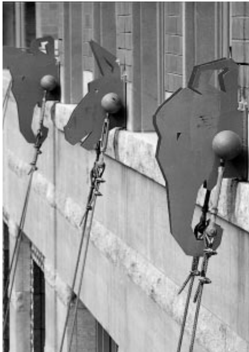
Contemporary laser cut steel figurative ornament is economical and reflective of contemporary technology. The donkeys and elephants embellish anchorage points for canopy cables. The subject matter reflects the particular interests of the building's occupants in Washington, D.C.
