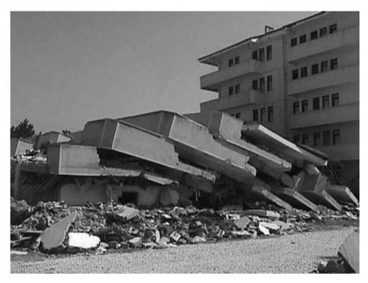
The photo, taken following the 1999 Izmit earthquake in Turkey, suggests that steel reinforcement in concrete columns and at junctions with floorslabs offered inadequate resistance to earthquake motion and to the load upon them. The collapsed floors remained largely intact. (Mehmet Celebi)
