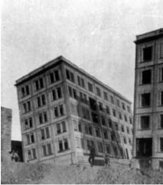
Fig. 5.12: Uneven settlement of building demonstrates monolithic strength of the Hennebique reinforced concrete construction system. Mill building, Tunisia, 1906. (Delhumeau et al.)
