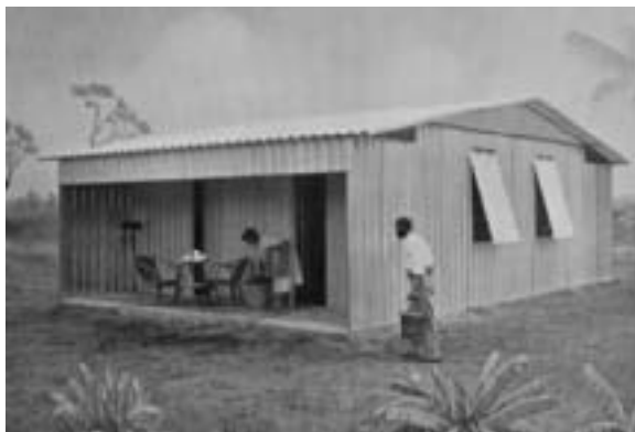
Fig. 3.1: Prefabricated aluminum house. The corrugated aluminum panels are both structure and environmental barrier. (London Northern Aluminum)
