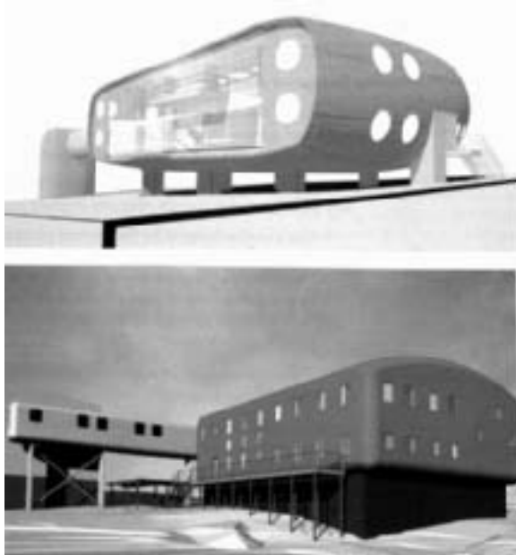
Fig. 4.6: Antarctic Station Design using FRP. Allen Jack + Cottier, 2003. (top) Competition entry. (bottom) Revised design. (Powell)
