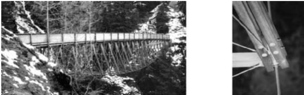
Fig. 4.8: Traversina Footbridge: elevation and strut detail. Jürg Conzett, engineer. Viamala, Graubünden, Switzerland. 1999. (Dooley)
