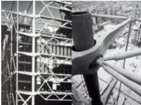
Fig. 5.5: Steel structural system of the Pompidou Center, Paris, Richard Rogers and Renzo Piano, architects, and Peter Rice of Ove Arup Ltd., engineer. 1976. (Rice)
