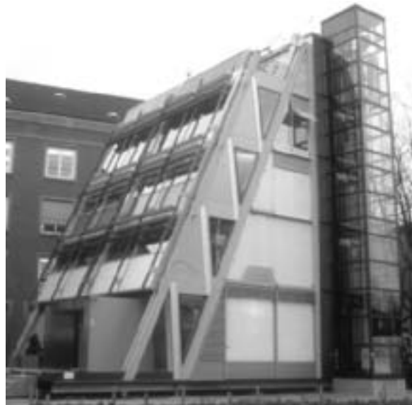
Fig. 6.31: Eyecatcher, Basel. Tallest all-FRP building at 5 stories. Artevelto Architects and CCLab, 1999.
