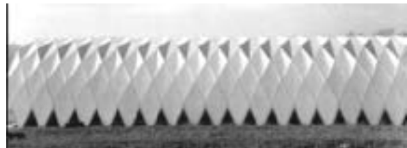
Fig. 6.10: Folded plate FRP vault structure for a sulfur factory in Rome. Renzo Piano, 1965. (Quarmby)
