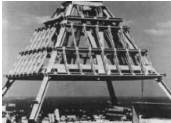
Fig. 6.24: Pultruded FRP structure of the Sun Bank turret, Orlando Florida, c.1990. (Chambers)
