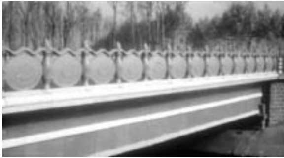
Fig. 6.16: Miyun Bridge, first all-FRP bridge in the world, China, 1982. (CCLab, after Meier)
