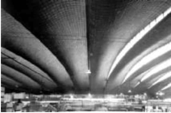
Fig. 4.32: Reinforced brick vault with Gaussian form. Citricos Caputto Packing Plant, Salto, Uruguay. Eladio Dieste, 1972. (Torrecillas)
