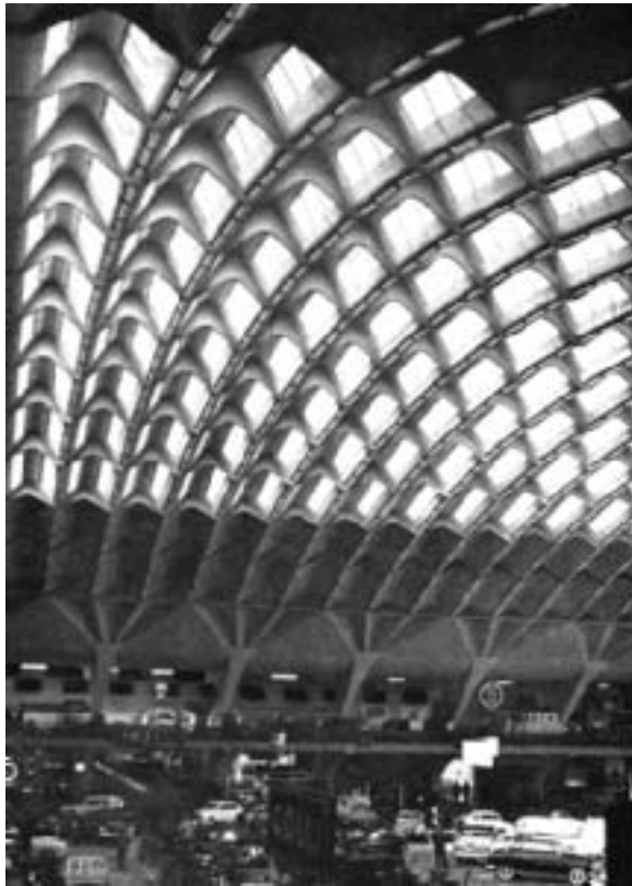
Fig. 5.8: Turin exposition hall. The vault is made from prefabricated ferro-cement segments 4.5 m long. Pier Luigi Nervi, 1947. (Desideri et al.)
