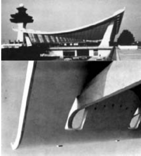
Fig. 5.9: General view and detail of cable suspended concrete roof of Dulles International Airport, Washington, D.C., Eero Saarinen, architect, Boyd G. Anderson, engineer. 1965. (Zannos)
