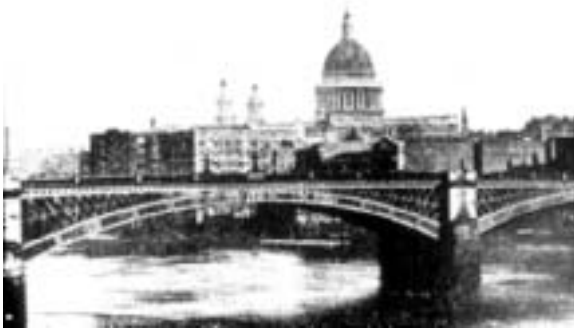
Fig. 5.13: Southwark Bridge, London. John Rennie, 1819. (Peters)
