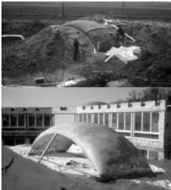
Fig. 4.24: Example of the hand lay-up method of producing complex FRP component. In this case the mold was formed with earth, however better quality can be attained in factory conditions.
