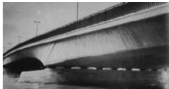
Fig. 4.11: Risorgimento Bridge, Verona, Italy. Pier Luigi Nervi, 1968. (Desideri et al.)
