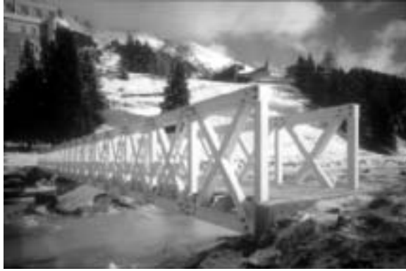
Fig. 6.22: All-FRP Pontresina Footbridge, Switzerland. CCLab, 1997. (CCLab)
