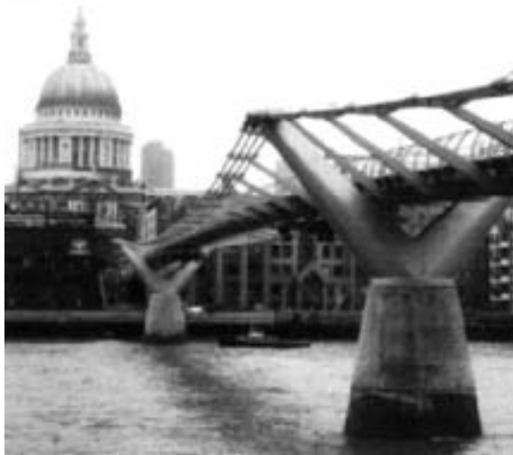
Fig. 4.7: Millennium Bridge, London. Norman Foster and Ove Arup & Partners, 2000. (Russell)
