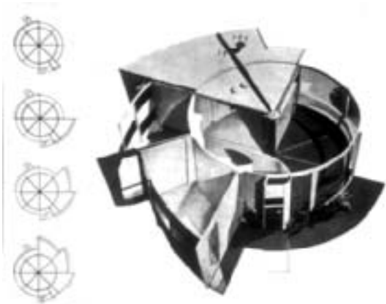
Fig. 6.7: First all-FRP house exhibited at Paris Exhibition of 1856. Ionel Schein, Yves Magnant, and R.A. Coulon. (Quarmby)
