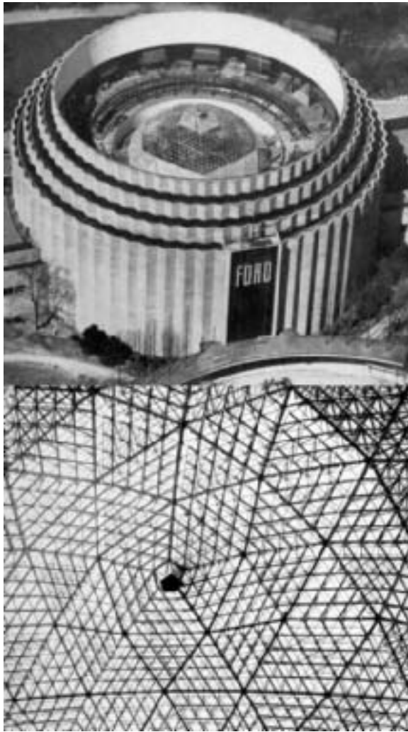
Fig. 4.38: Geodesic dome of the Ford Motor Company's headquarters, Dearborn Michigan. Diameter = 31 m, weight = 8.5 tons. Buckminster Fuller, 1953. (Peter)
