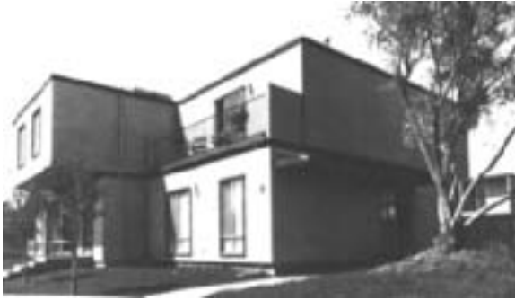
Fig. 6.11: Filament wound, FRP low-cost housing unit, USA. TRW Systems, 1968-1973. (CCLab)
