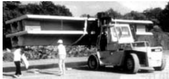
Fig. 6.20: All-FRP Smith Road Bridge, USA. Martin Marietta Materials, 1997. (CCLab, after Martin Marietta)
