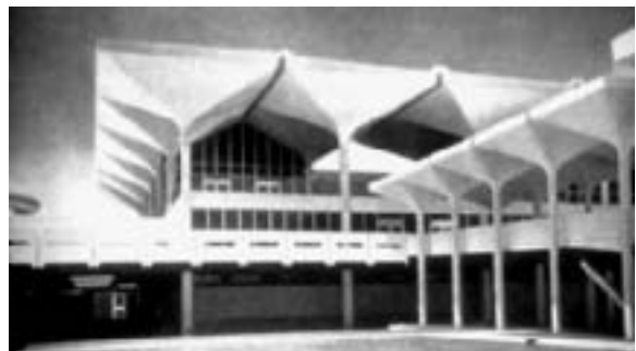
Fig. 6.15: FRP roof of Dubai Airport, United Arab Emirates. Pae & Broughton, 1972. (CCLab)
