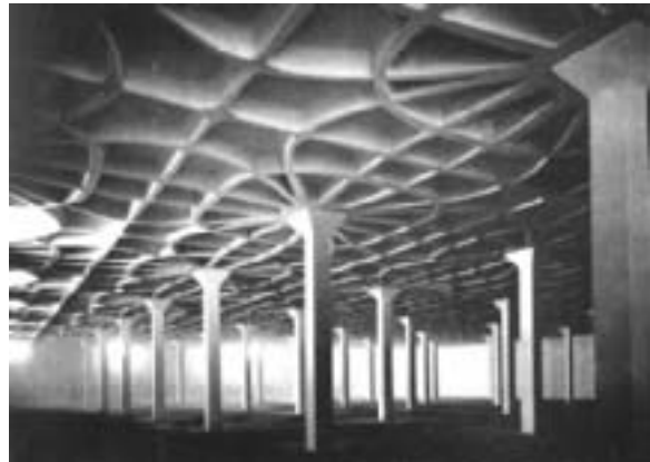
Fig. 5.7: Underside of floor slab of the Gatti wool factory showing isostatic stress lines, Rome, Pier Luigi Nervi. 1951. (Nervi 2 )
