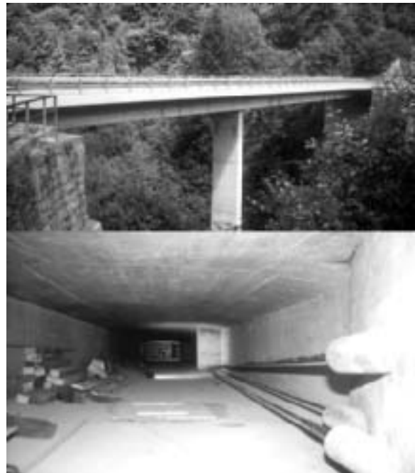
Fig. 6.21: CFRP cable strengthening of Verdasio Bridge, Switzerland. CCLab, 1999. (CCLab)
