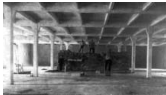
Fig. 5.11: View of Hennebique reinforced concrete construction system. Warehouse in Nantes, France. Clériceau and Tessier, architects, 1903. (Delhumeau et al.)
