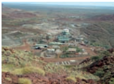
Wodgina processing plant
