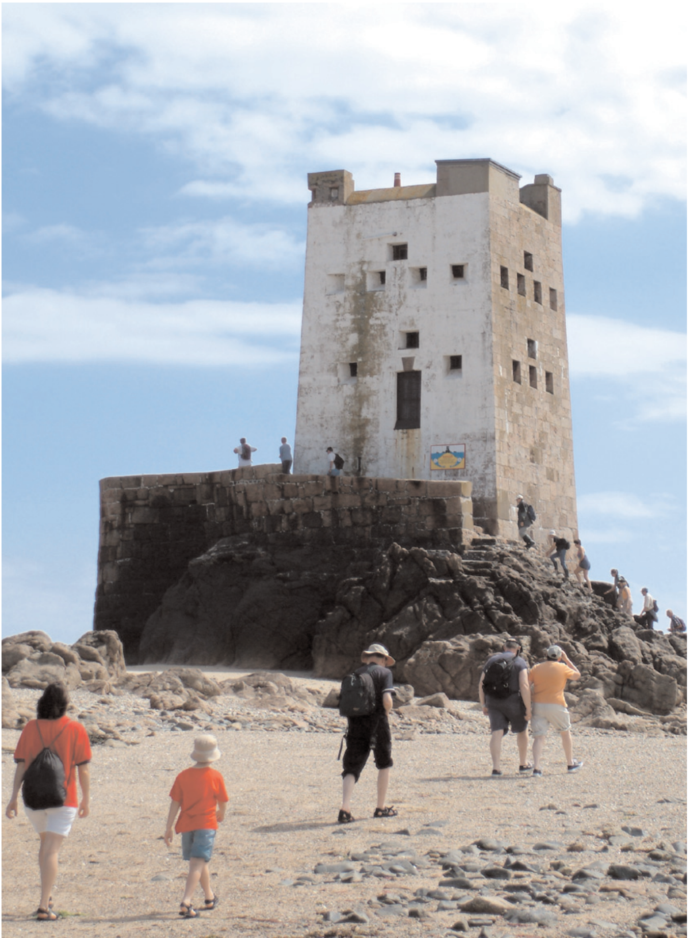
Seymour Tower, built in the late 18th century to repel French invaders, stands two kilometres offshore in the middle of one of Europe's largest intertidal reef sites. Tides here can recede almost four kilometres from shore.
