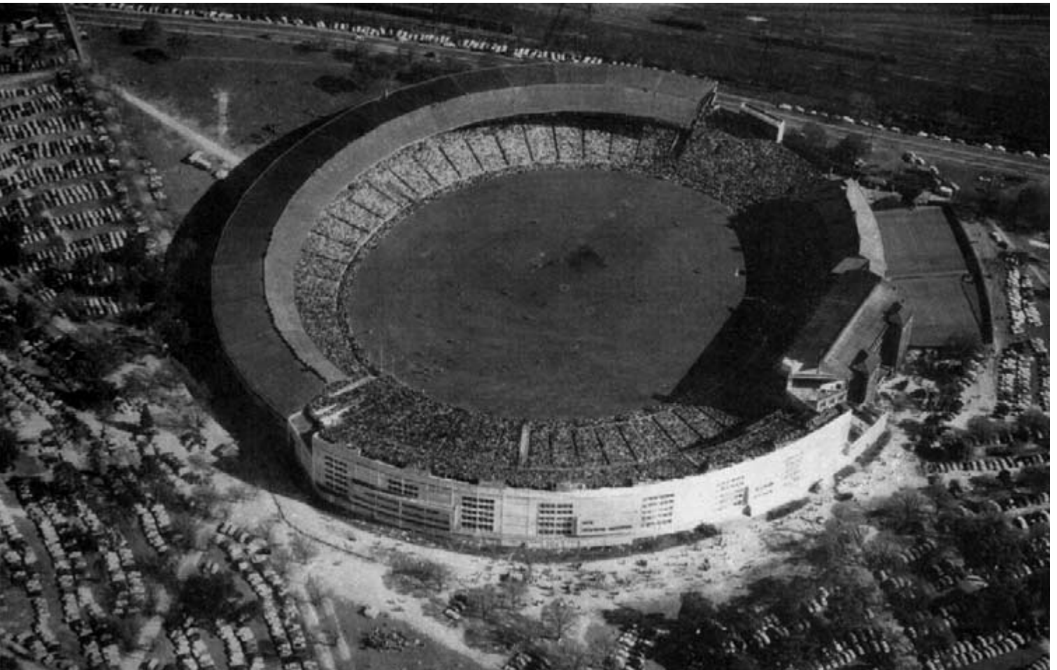
The Main Stadium prior to track being laid.
