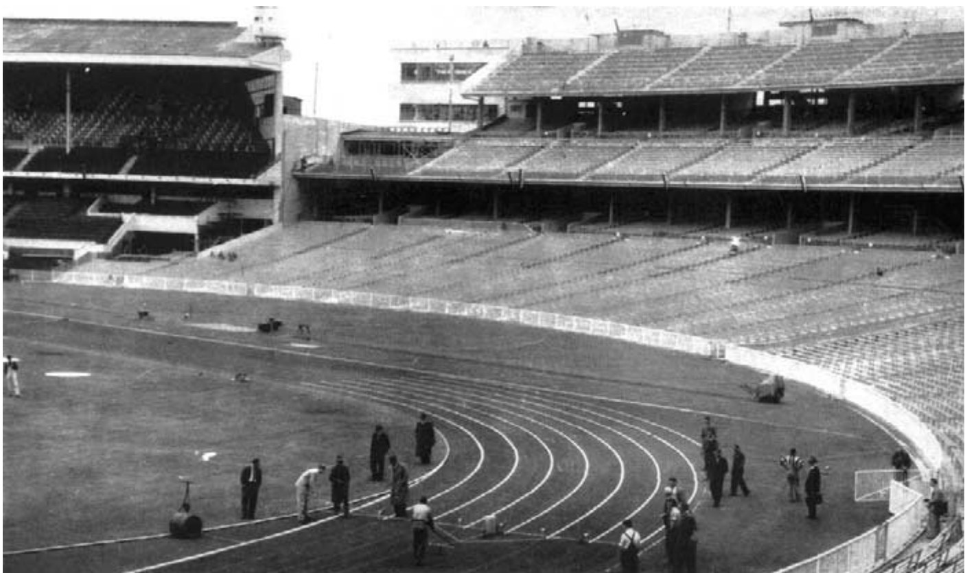
The 8-lane marking machine in operation.
