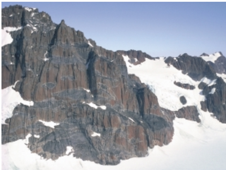
Fig. 14. Upper part of the 1740 Ma post-tectonic Graah Fjelde rapakivi granite intrusion, with large rafts of older Ketilidian country rocks (dark grey). Outer coastal area north of Danell Fjord (c. 61°N), South-East Greenland; the exposure is c. 600 m high. Photo: A.A. Garde.
