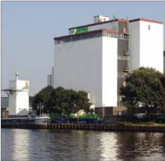
De Heus Voeders broiler feed mill in Meppel, Netherlands.
