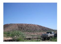
There is now a strong movement to invest in methods of rainfall harvesting and storage. We saw 30 ha man-made catchments where they have built contoured, graded, water-collecting pads that allow harvested water to run to a dam with a turkey nest ('Tanque Australiano') which is used to distribute water by underground plastic pipes to troughs across the property
