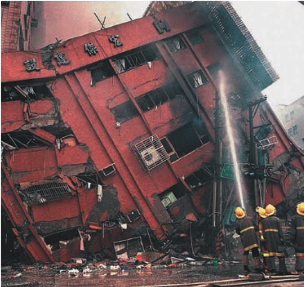
SEVERE DAMAGE CAUSED BY THE TAIWAN EARTHQUAKE, SEPTEMBER 1999.
