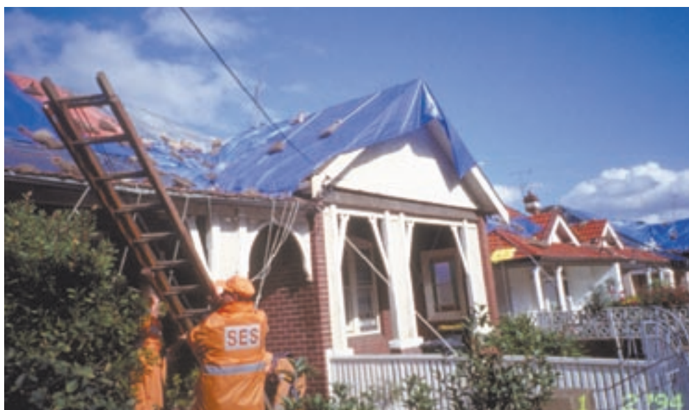
REPAIRING SEVERE STORM DAMAGE, SYDNEY, APRIL 1999.
