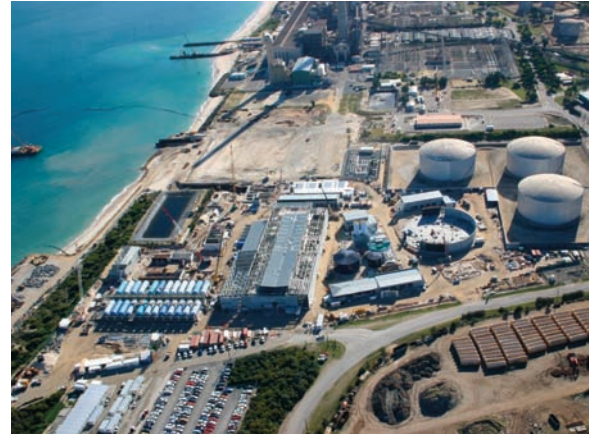
Aerial view of the Perth Desalination Plant in Kwinana, Western Australia.
