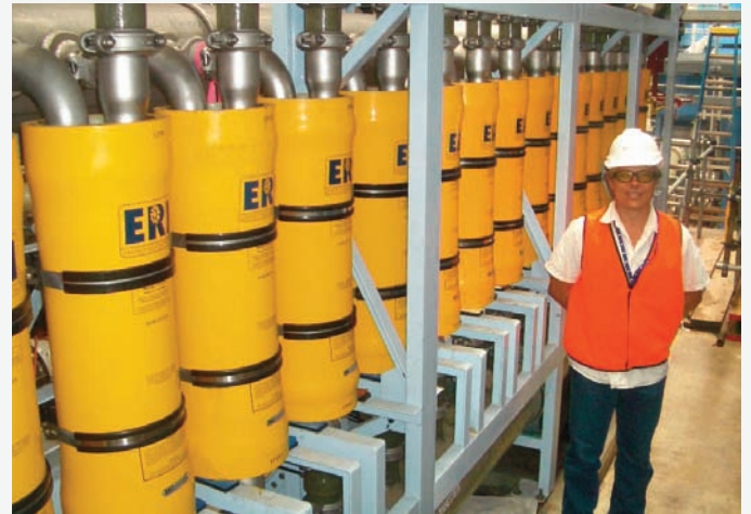
Gary Crisp stands by the first of 12 SWRO train of 16—PX-220 Pressure Exchangers.
